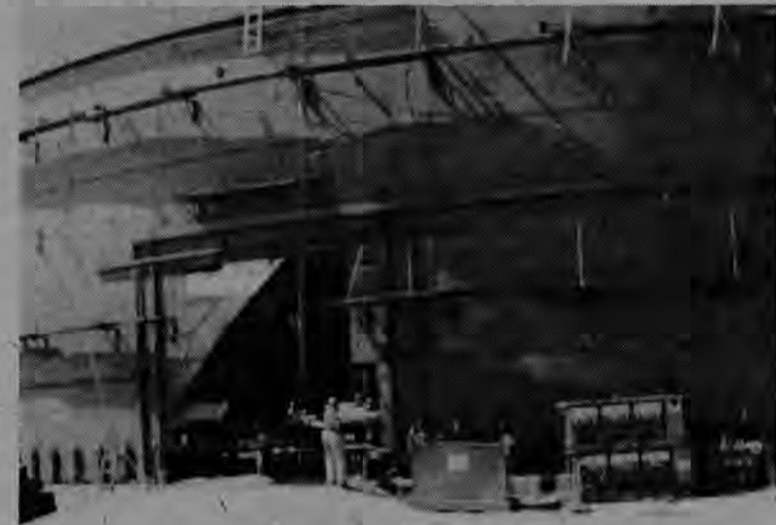
Six miles north of Lovelock, Local 3 members are helping to construct a one million barrel LNG storage tank for Southwest Gas Company. The tank measures 185 feet in diameter, 80 feet high and is being built by Chicago Bridge and Iron.
