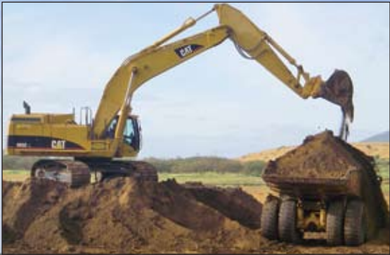
Operators Malcolm Park and Gilbert Kahaleauki Jr. haul backfill material for a 96-inch cap-corrugated, aluminum-pipe drain-line.
