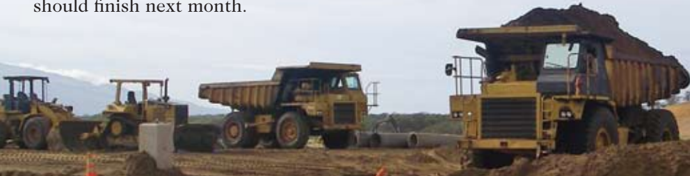
Operators Malcolm Park and Gilbert Kahaleauki Jr. haul backfill material for a 96-inch cap-corrugated, aluminum-pipe drain-line.
