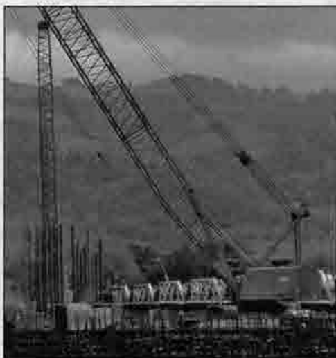
After the footings of this bridge in Geyserville failed due to December rains, members for Foundation Construction began repairs on Hwy. 128.
