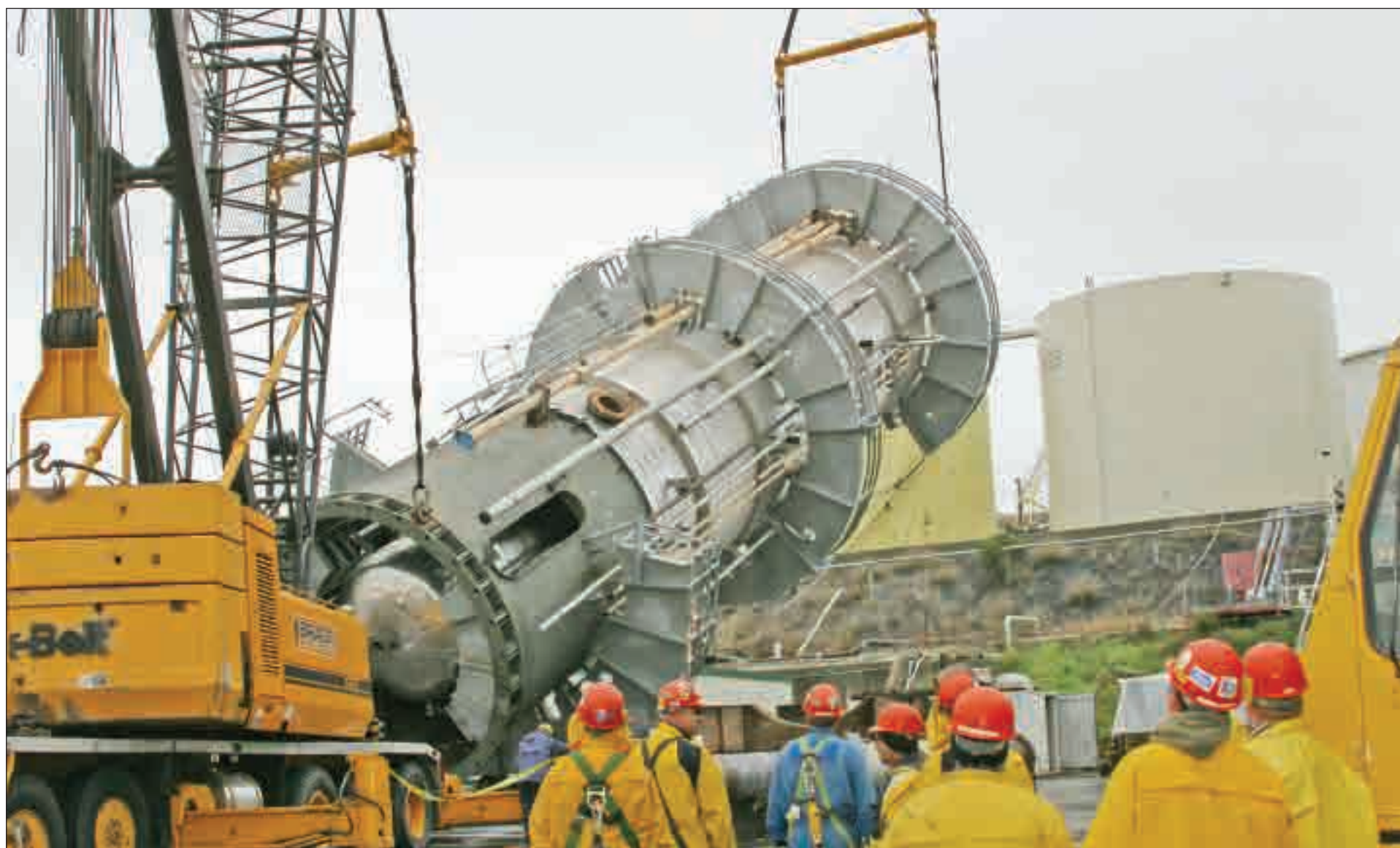
Local 3 workers look on as the vacuum tower is up-ended by two cranes.
