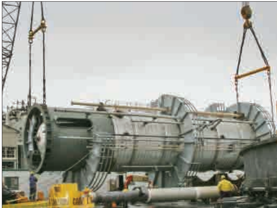
Two cranes, operated by Local 3's Randy Fall and Brian Casjens, up-end this fractionalization tower and move it to its desired location at the ConocoPhillips refinery in Rodeo.
