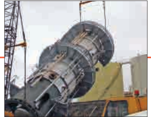
The ConocoPhillips vacuum tower is up-ended by Local 3 crane operators Randy Fall and Brian Casjens..... 9
