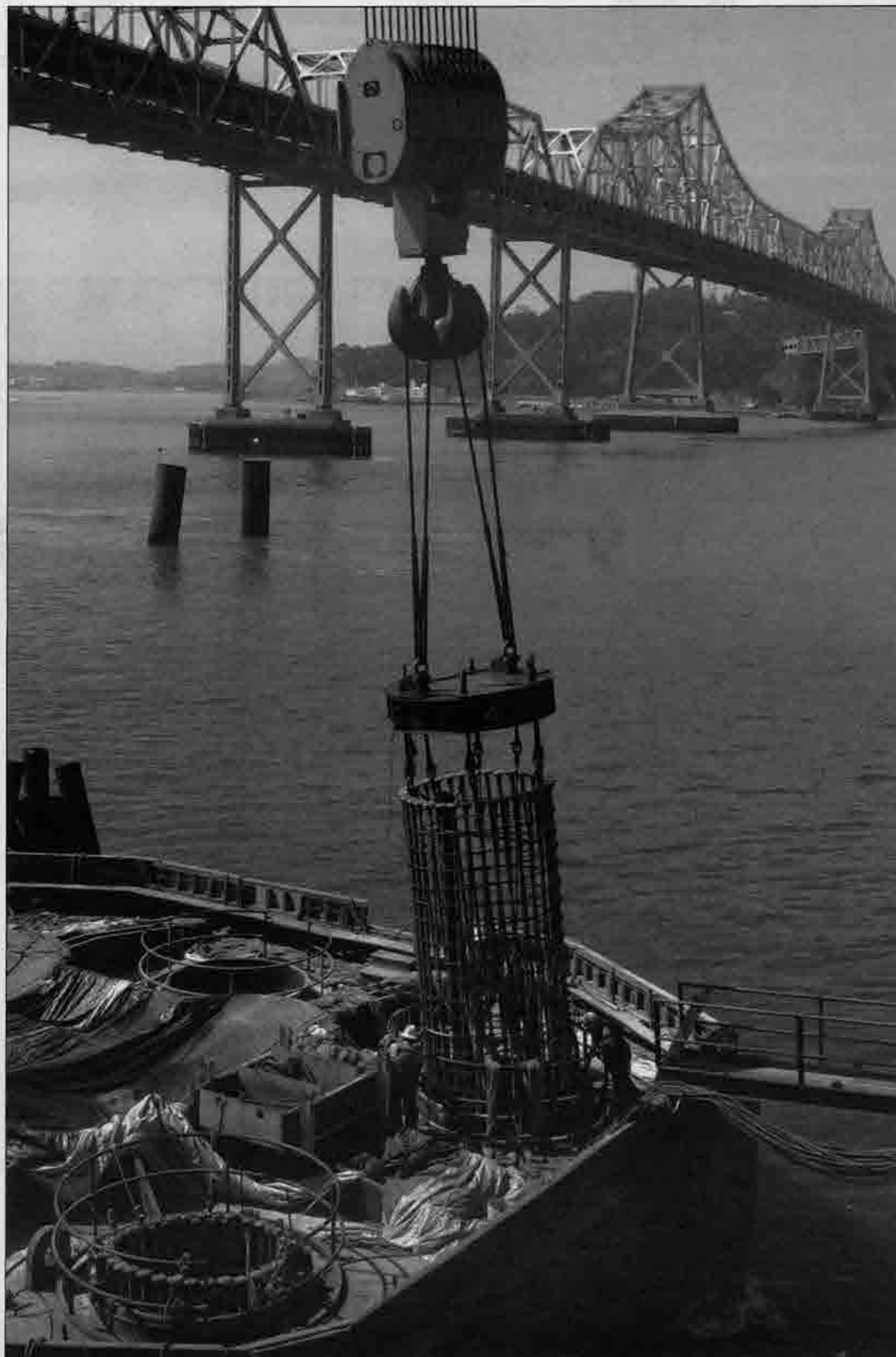
A 160-foot rebar cage is set into driven pile on Pier 7.
