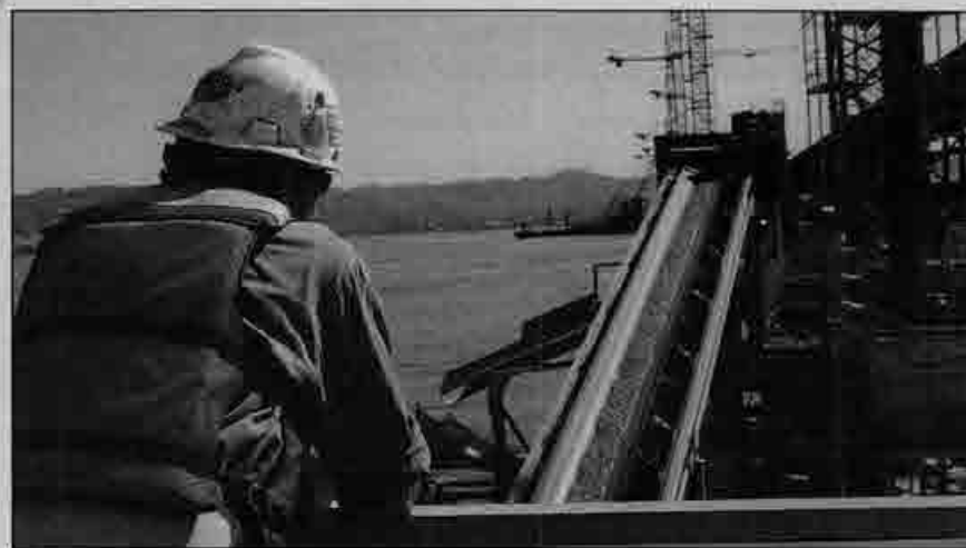
Barge Engineer and Captain James Lavell, a 23-year Local 3 member, monitors the concrete as it is carried up the 50-foot conveyor belt and into the hopper, which then shakes it into the remixer.
