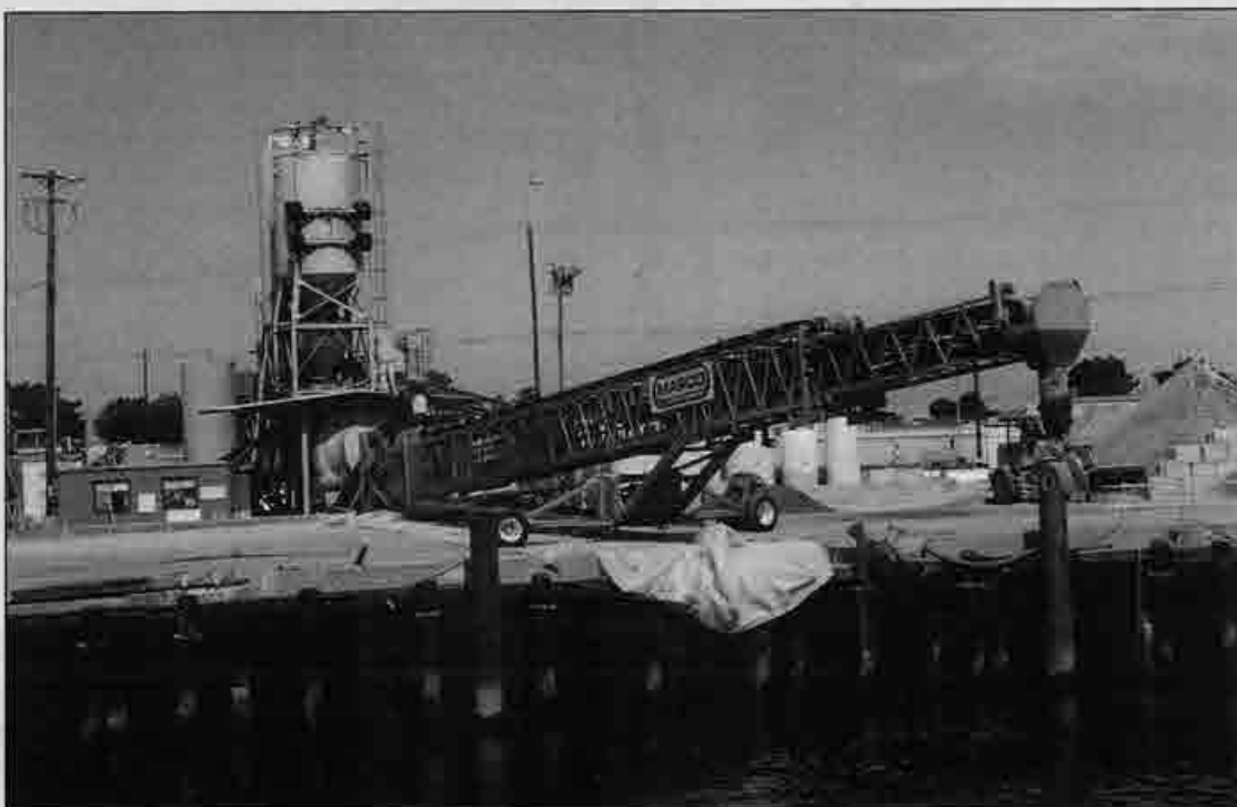
The concrete batch plant is positioned next to the San Francisco Bay so that concrete barges can load up the newly mixed concrete and take it to the bridge jobsite. A conveyor loads the concrete from the batch plant into the mixer on the barge.
