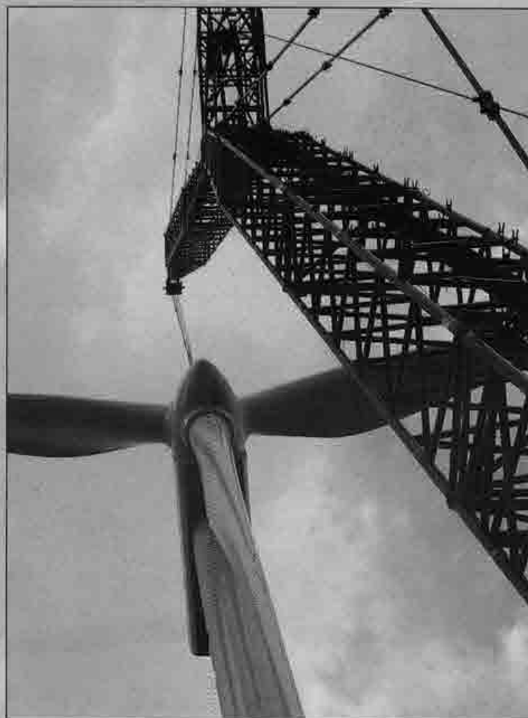
The crane keeps the rotor steady as it is bolted in place.
