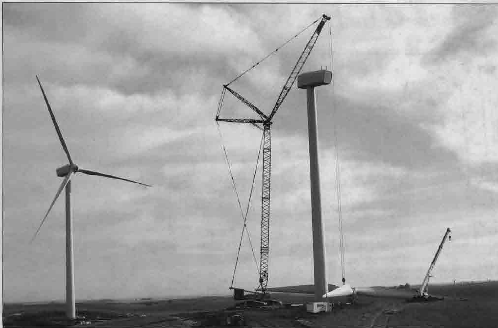
The crew prepares to lift the rotor onto the nacelle.
