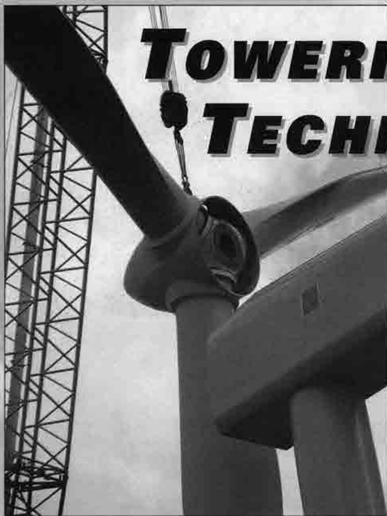
The rotor is lowered to the nacelle.
