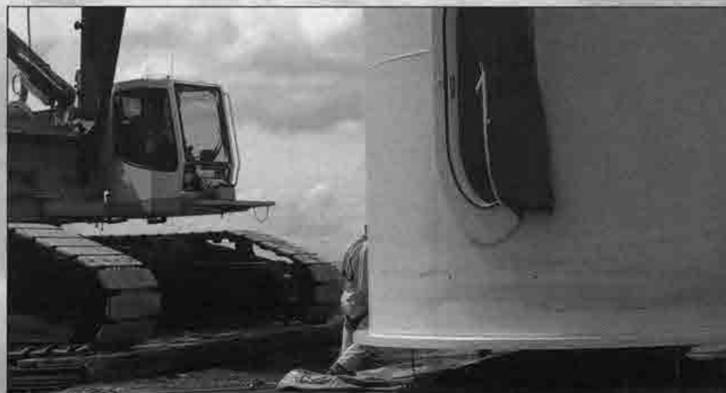
Operator Bob Lohr prepares to lower the base section of the tower onto its foundation.
