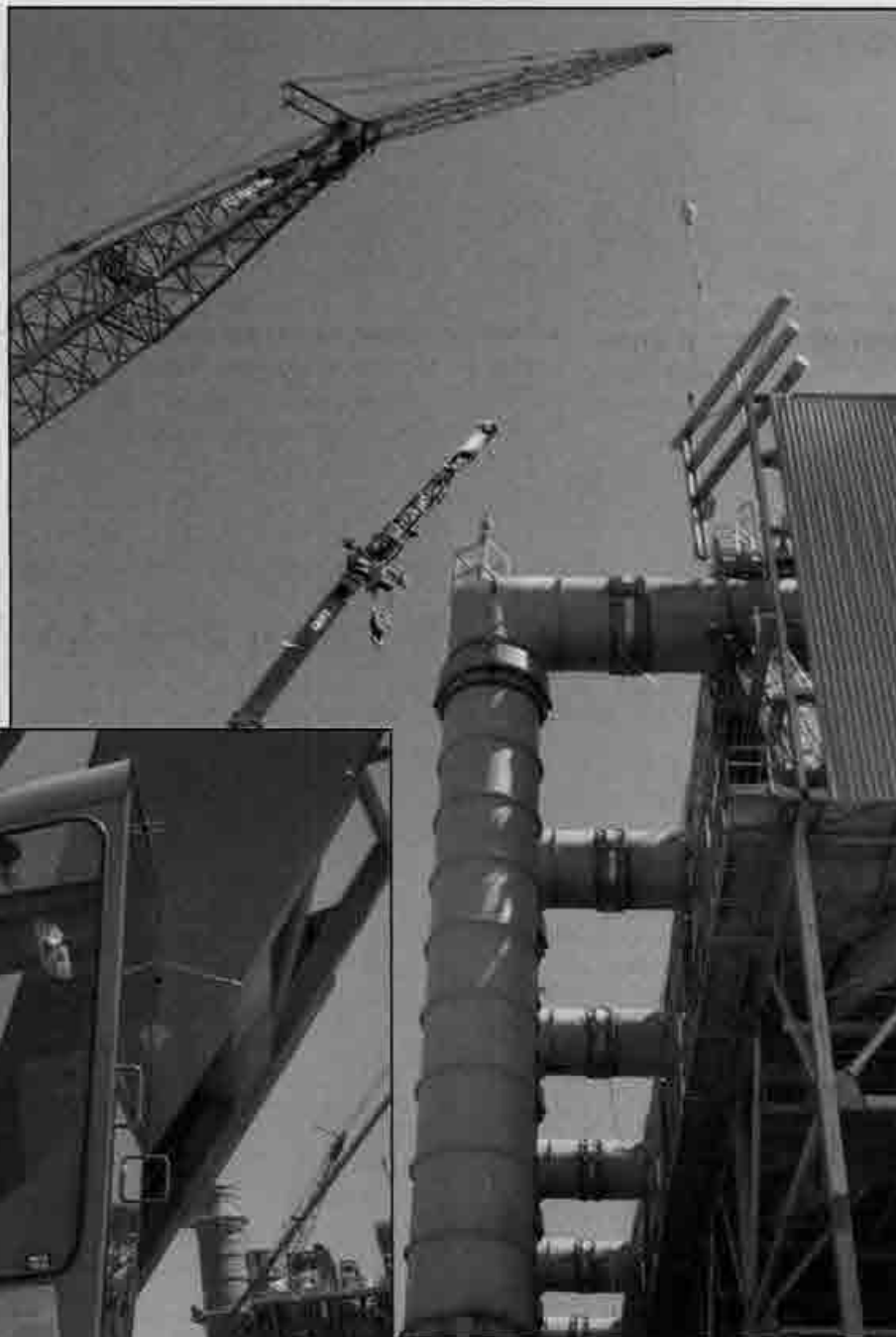
With help from Local 3 membership, the final structural arm for the cooling tower complex at Calpine's power plant southwest of Yuba City is lowered into place.
