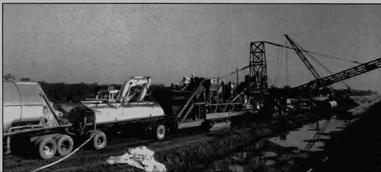
▲ Mountain Cascade's soil processor at work on Modesto Irrigation District's 16-mile water pipeline project.
