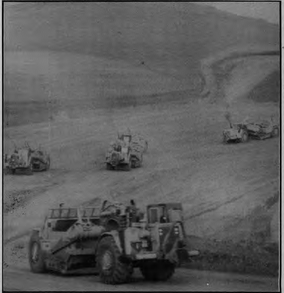
Above: Ferma has about 40 scrapers moving 50,000 yards a day from a cut to this fill area.
