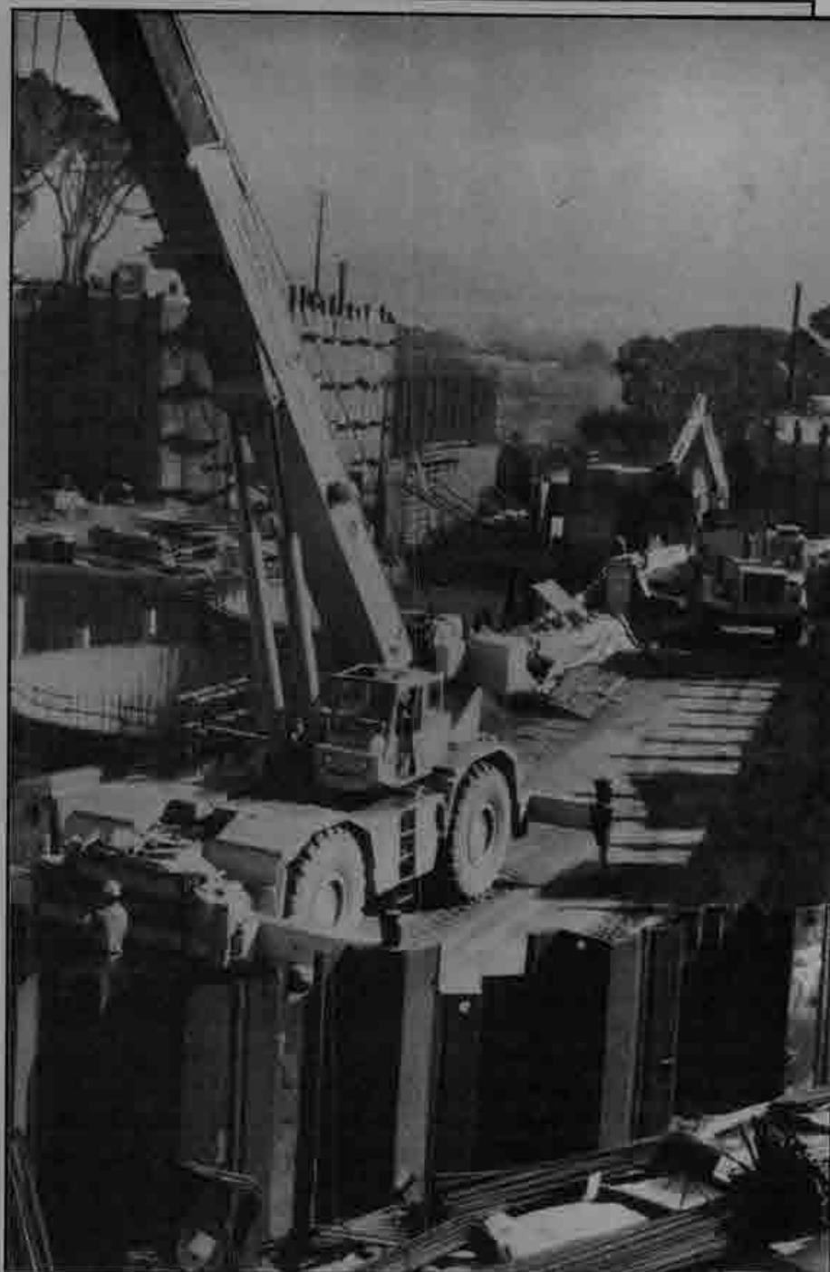
Above right: One of the 12 cranes on the job lifts pieces of rebar into place while a backhoe and loader work on trenching for pipelines and utilities.
