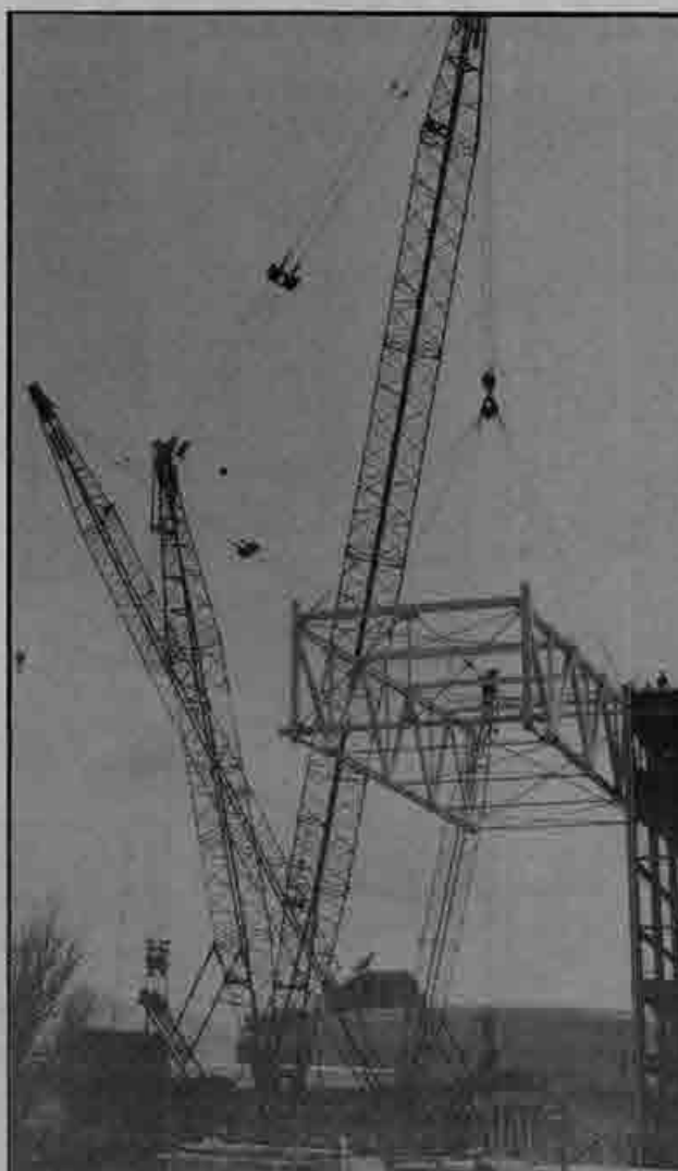
A 4100 Manitowac hoists one of the 10 trusses being installed on top of the new Utah Jazz basketball arena.
