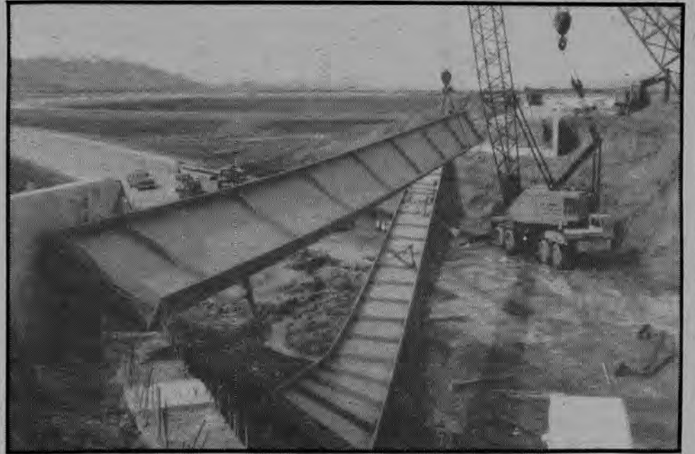
Quick thinking on the part of the operators and workers below saved some injuries on this I-80 mishap in Salt Lake when a strong gust of wind blew two beams on an overpass job.
