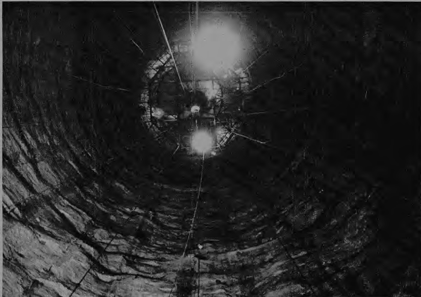
Looking up the T-3 Surge Chamber at the Helms project, the entrance to the shaft 500 feet up is barely visible.
