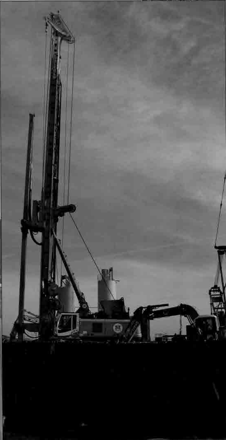
Danny Boswell operates the BG40 drill on the Alternative Intake project, drilling more than 100 feet down, as Catherine "Earl" Lytle removes dirt with a mini excavator.
