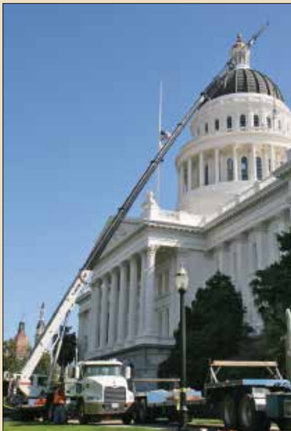
With 230 feet of boom, Ron Shoffit works with precision to hoist the steel up to the rotunda.
