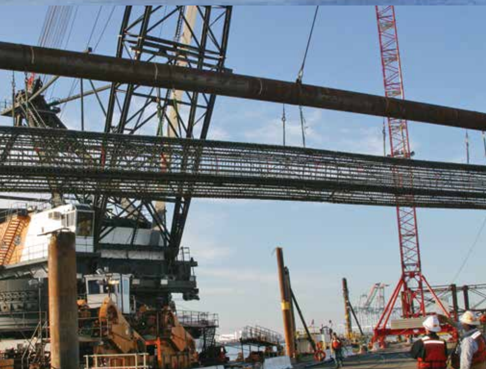
The Derrick Barge (DB) General slowly swivels around to place one of the last rebar cages from the KFM yard onto an awaiting barge. The crew running the General includes Operator Tim Lassiter and deck engineers Tom Butcher, Keith Lassiter and Ronnie Robinson.
