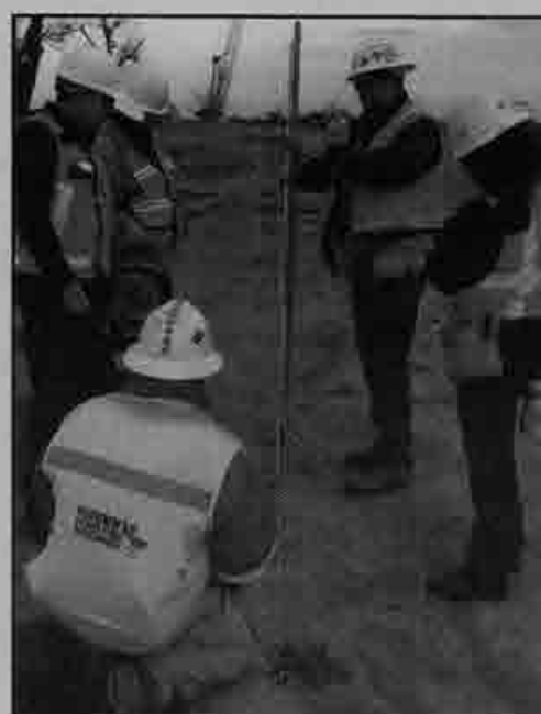
Left to Right: Denis Monzon, instructor; Gary Pyron; Jon Evans holding rule; Misty Costa; Tom Zenahlik kneeling. Trainees aligning stakes getting ready to measure for hike-ups.
