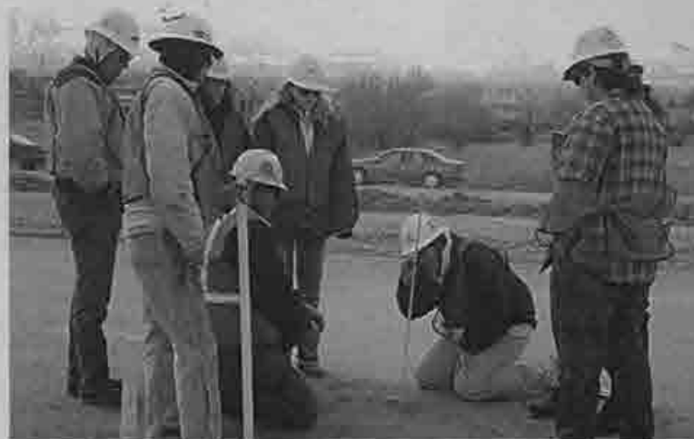
General foreman Gerald Zorr works with group on shooting grade and reading stakes.
