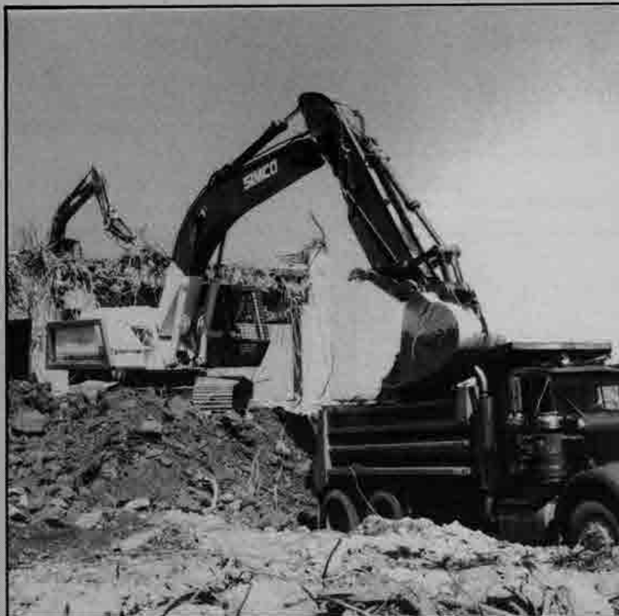
The structure's 60,000 cubic yards of concrete is being hauled to a crusher in an estimated 5,000 to 6,000 dump truck loads.
