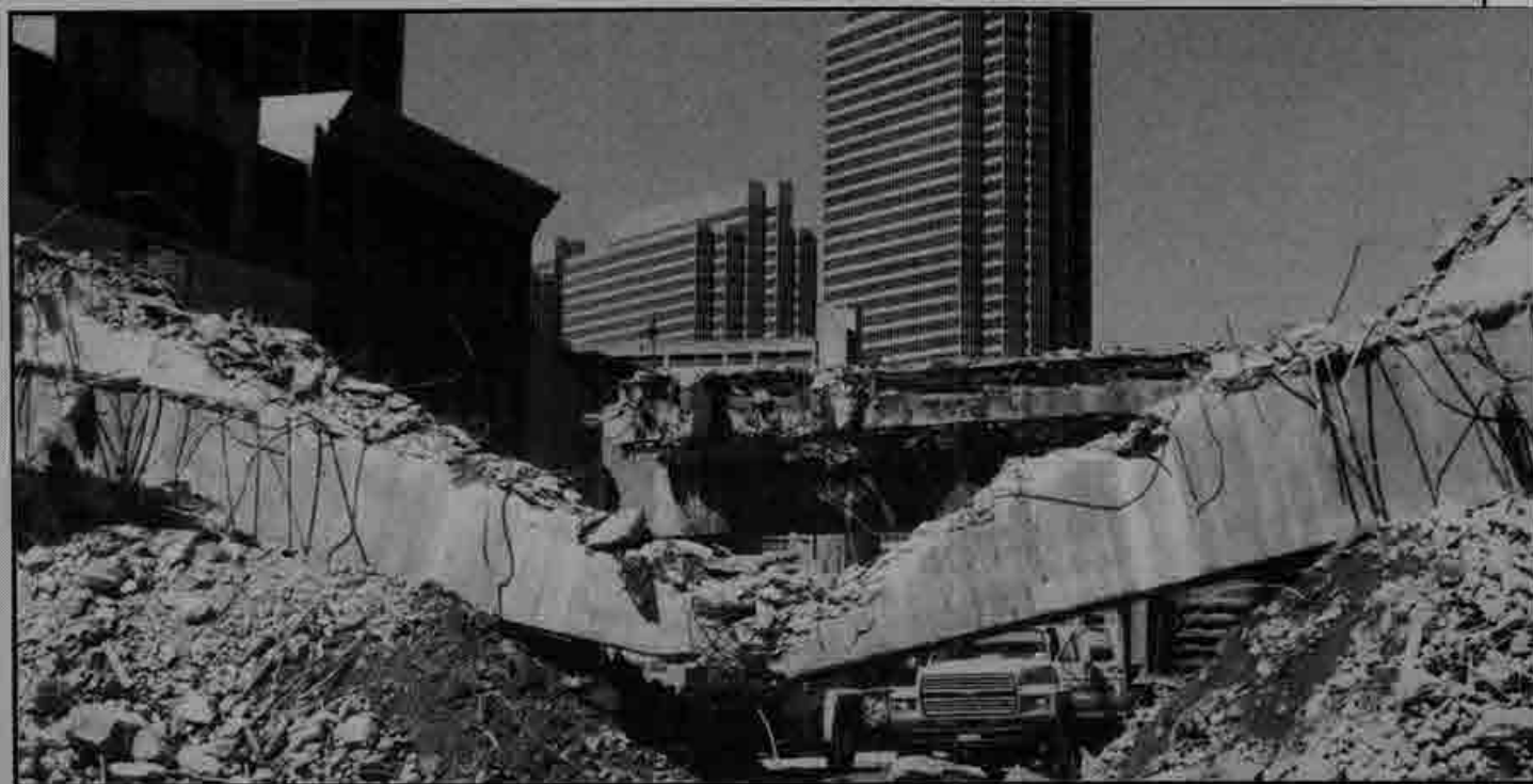
The transverse bents are chiseled away in a half-moon pattern so they buckle inward instead of collapsing outward onto the street.
