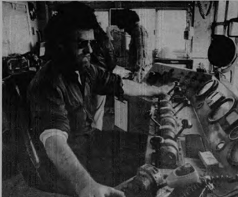
Leverman Jack Tuttle (above) keeps his eye on the gauges of Shellmaker's suction dredge, as the rig cuts a 300-ft. swath along the river channel next to Venice Island. Material is deposited on the other side of the levee (upper left).
