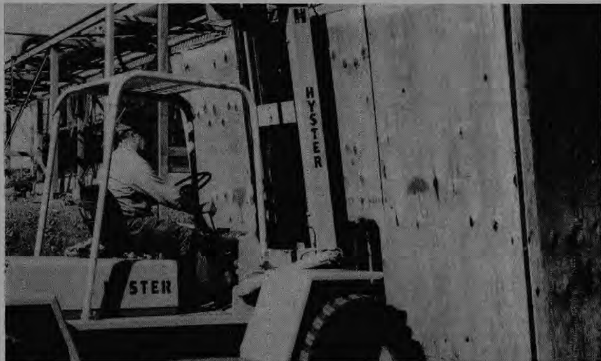
Brother Tommy Rapoza unloads crates on the HGP-A Geothermal Project.
