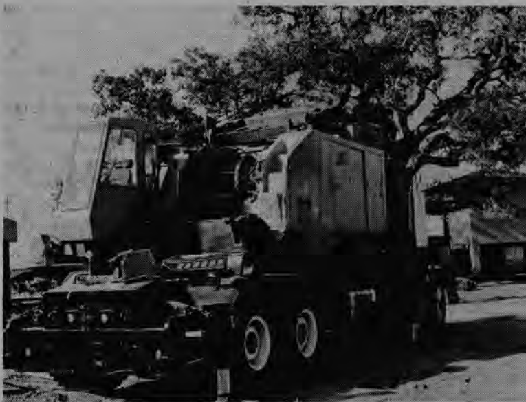
Pictured above is a 150-ton American truck crane which suffered a collapsed boom on a modular condominium development complex in San Jose. The boom was completely
