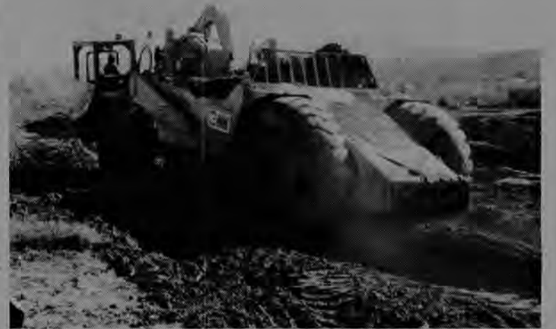
Local 3 member Jack Carson operates CAT 631 scraper on the Humboldt River Relocation Project—part of the two-year long railroad relocation project near Elko, Nevada.
