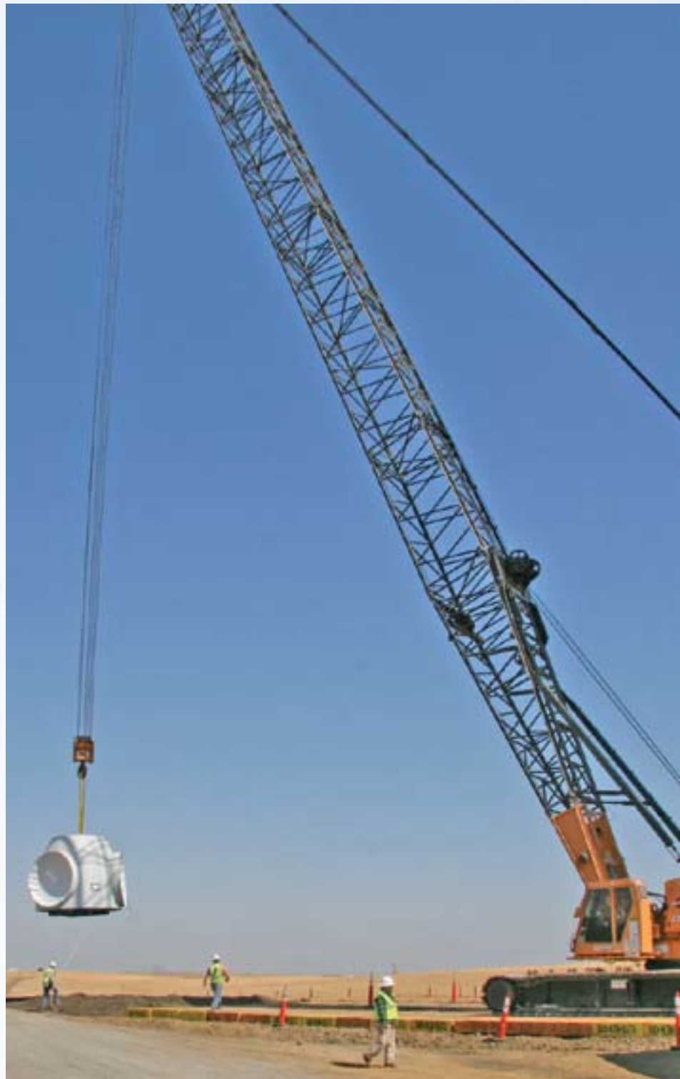
Bragg Crane Operator Calvin Bottolfson lifts the hub for one of 75 wind turbines erected for the Shiloh II job.
