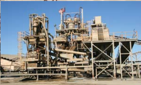
The mineral or "jig" tower washes the rock after it is mined at the Teichert Aggregates Plant in Marysville.
