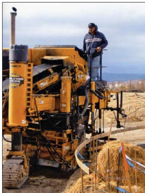
Member David Muñoz Caro operates a curb and gutter machine at Fellin Road in Dublin for Murga, Strange and Chalmers.
