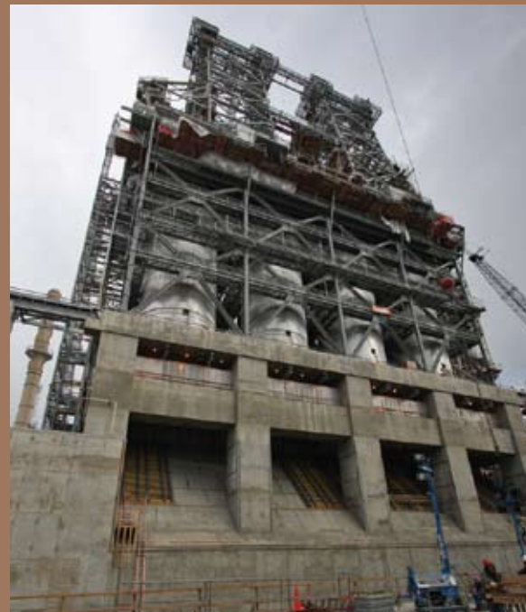
The concrete pour for the base of the coker plant shown here took 775 truckloads of concrete and lasted 23 hours straight.
