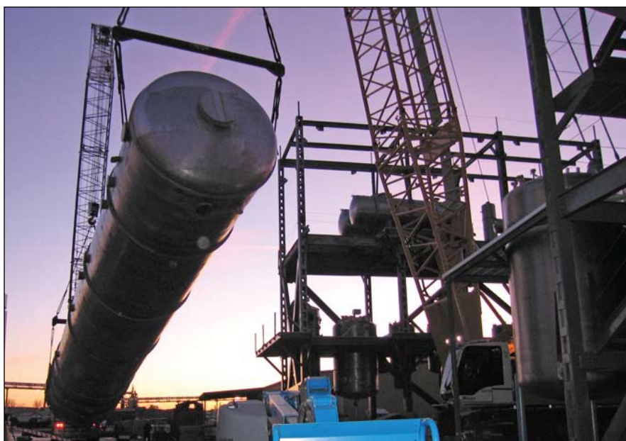
Crane Operator Steve Faughnan and Oiler Chris Christy work together with Crane Operator Adam O'Brian and Oiler Adam Mitchell to lift two 280,000-pound tanks at the Keys Ethanol Plant.
