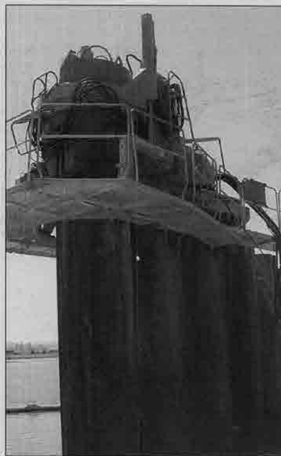
The Giken pile-driver uses hydraulic-press technology to silently drive pile.
