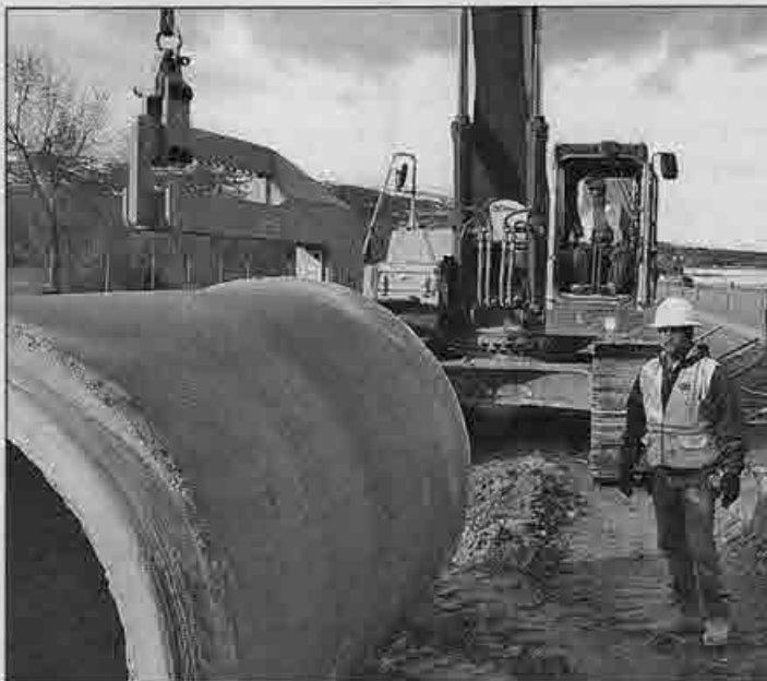
Local 3 members Gary Bitz and Robert Sanchez set a 53-inch drainage pipe on the Moana Lane Project.
