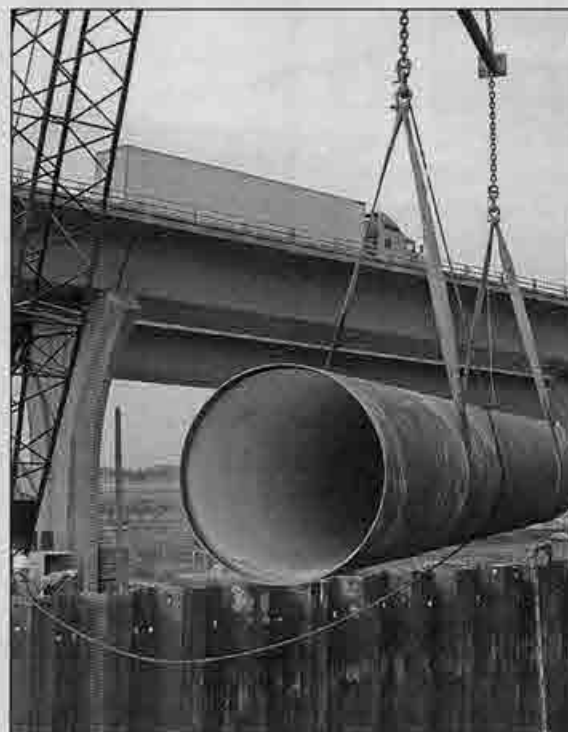
Crane Operator Jimmy Jacobs lowers a section of pipe down to crew members 40 feet below.
