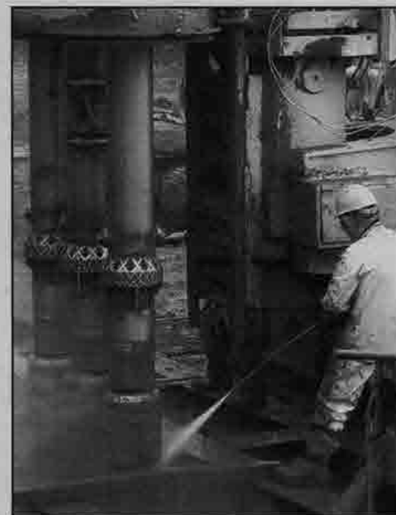
CLEAN CUT: Local 3 member Gary Johnson steam cleans mud and debris from Raito's triple-auger Dynamic Hercules 808 rig. "That way dirt don't fall on you," fellow Operating Engineer Chris Johnson said.
