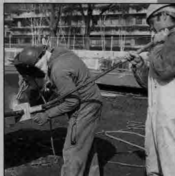
TEAMWORK: Chris Johnson, right, a member of Local 3 for six years, braces a steel sheet pile for welder Buzz Kelley, a five-year member of Local 3. The 50-foot-long, 4,800-pound sheet piles are lowered into the ground to support a 2,100-foot reinforcing wall.
