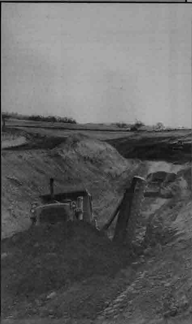
Right: Dozer Operator Don Mitchell shapes a section of the canal.
