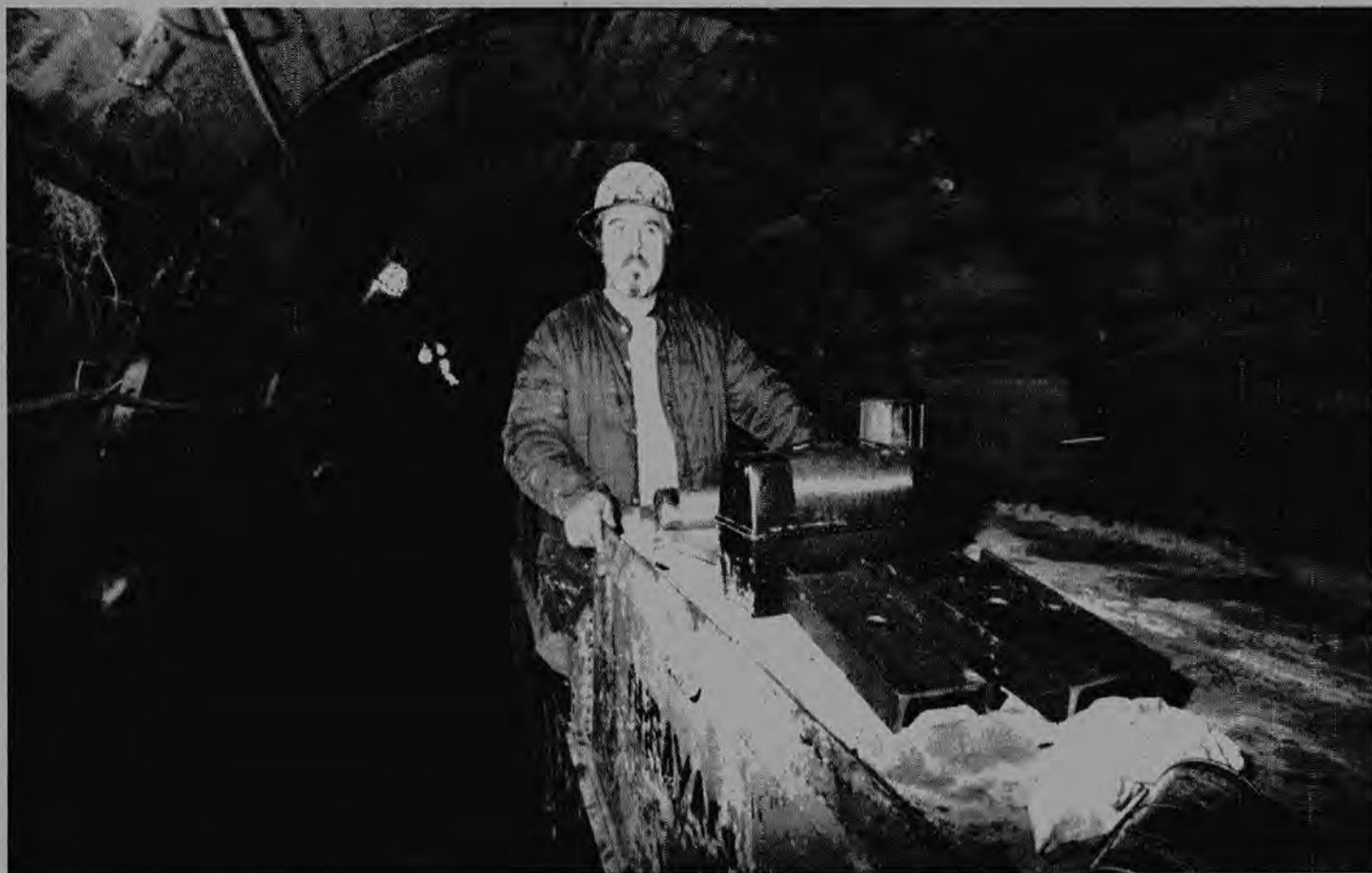
Pictured top left, Local 3 member Don Rush operates a tunnel locomotive used in transporting the cement agitator on the N-1 side of the tunnel.
