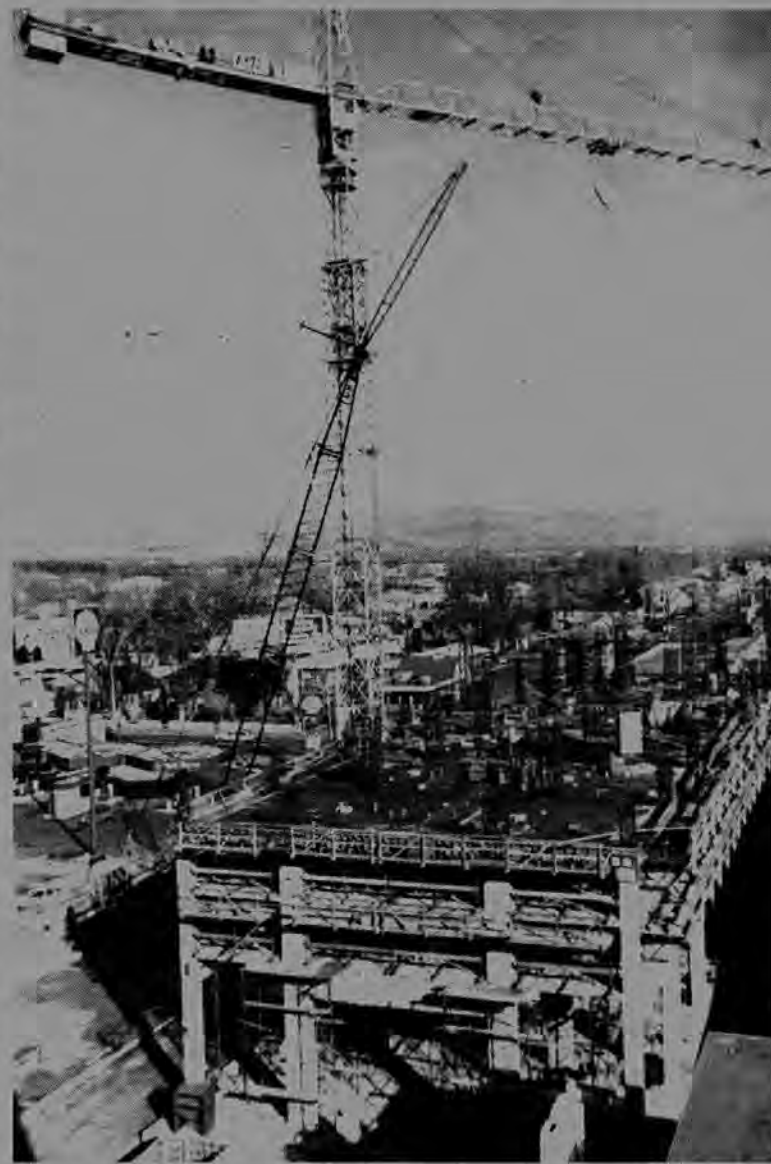
Pictured above are the two cranes currently working on the 22-story Circus-Circus Tower project in Reno.
