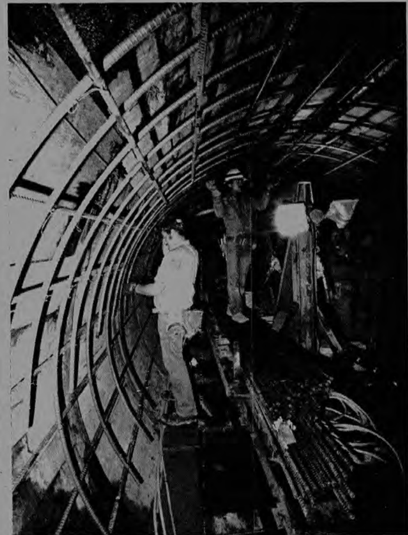
Pictured top right are Local 3 leadman Marc Seaford and heavy duty repairman Gary DeRenzi tying off a barrel to be lifted from the shaft of N-2. Pictured immediately above are ironworkers placing rebar on the N-1 side of the tunnel.
