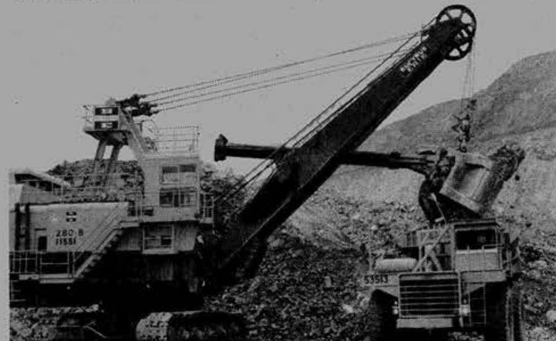
PICTURED ABOVE is the specially designed 280-B shovel which is currently working two shifts at New Melones Dam site. Below is a view of the fill area of the earth dam. The fill is about one third completed, according to supervisors on the job.
