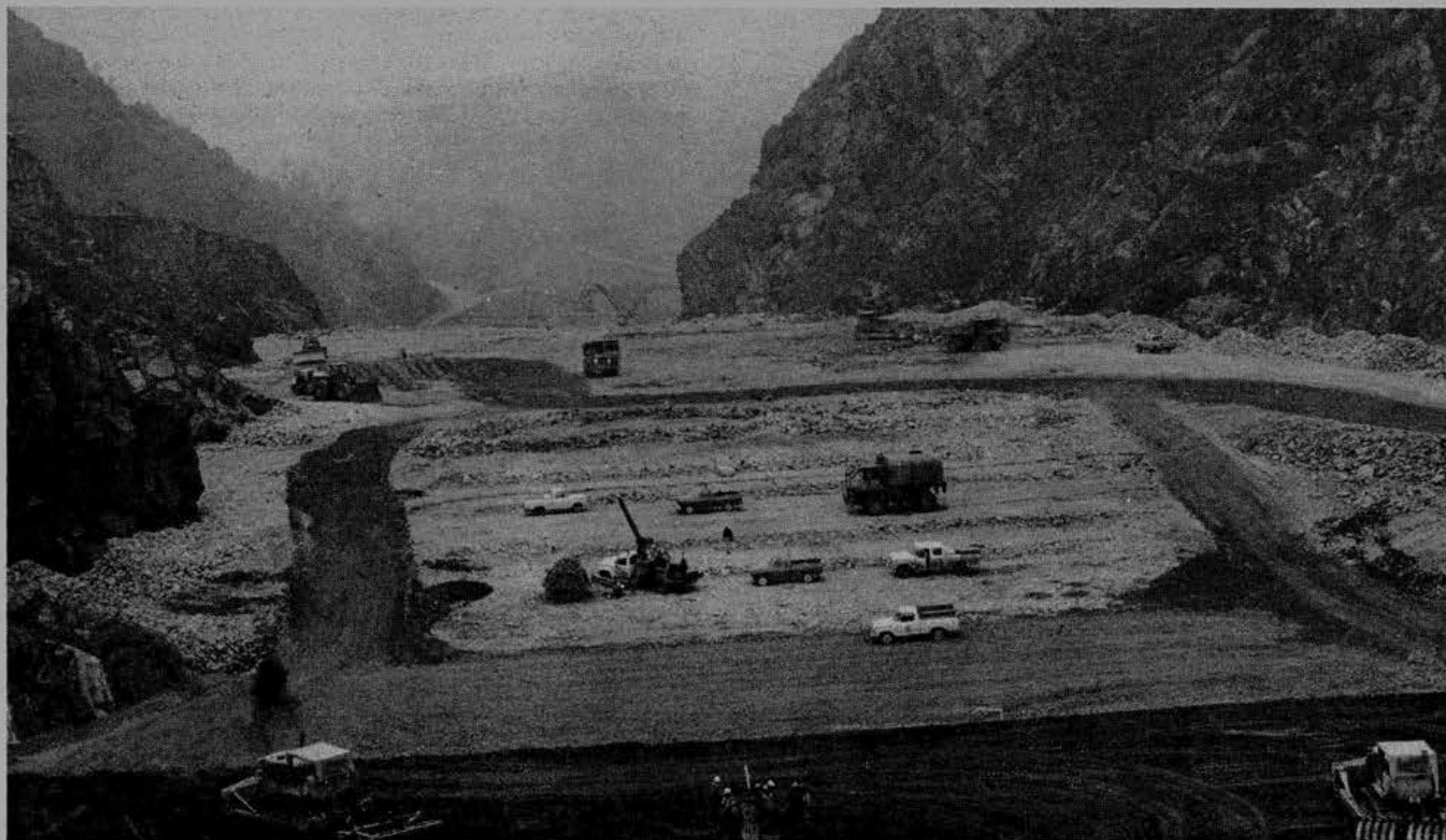
PICTURED ABOVE is the specially designed 280-B shovel which is currently working two shifts at New Melones Dam site. Below is a view of the fill area of the earth dam. The fill is about one third completed, according to supervisors on the job.
