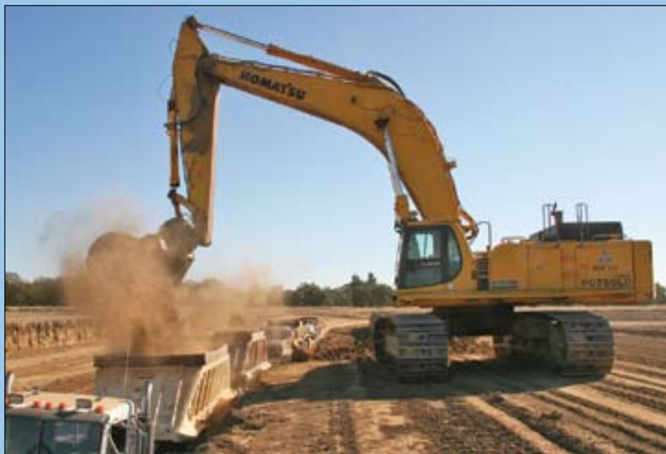
Excavator Operator Jon Lovell loads trucks with dirt extracted from the Platter Borrow Pit, one of many borrow pits on the Feather River Setback Levee project.
