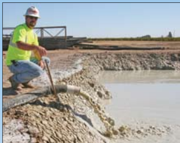
Guy Adams, a 12-year Local 3 member, oversees the mixing of betinite, the material that will line the new levee.
