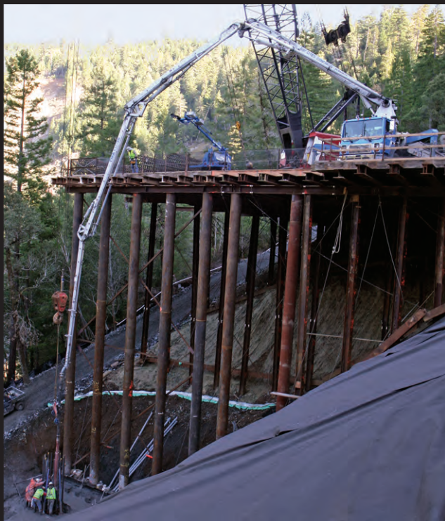
ON THE COVER: Pacific Coast Drilling Co. and Bay Cities Concrete Pumping work together to put in a pier for the new south bridge at Confusion Hill.
