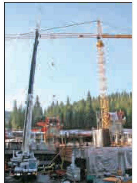
From left: Working in tandem at the Village at Northstar Project, seven-year member Matt Dunlap operates the Hydro 70-ton crane and 20-year member Ricardo Fernandez runs Crane Two, a Liebherr 316 EC-H12.
