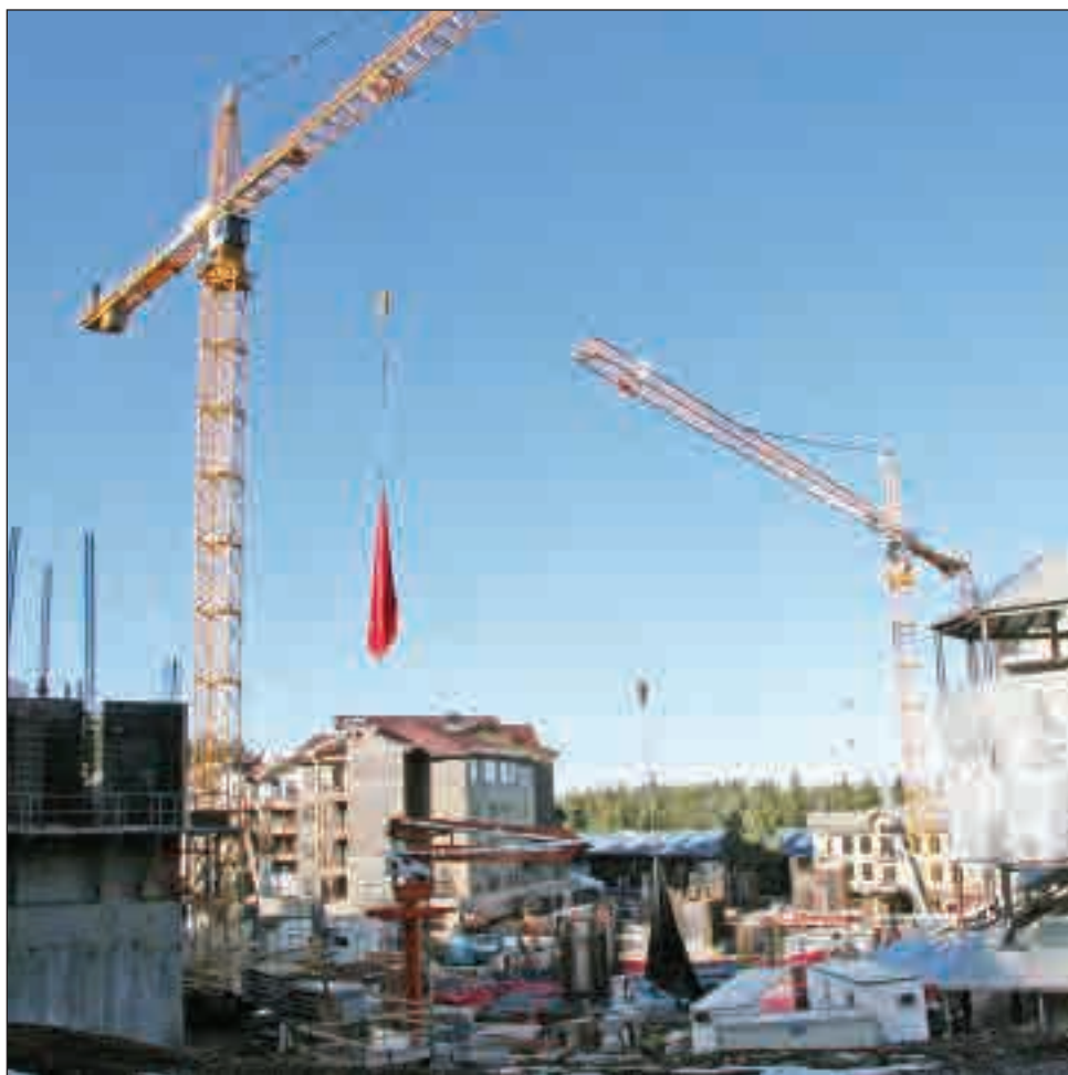
At the end of the workday, operators cover the rebar mat in blankets to prevent it from being covered in snow. The blankets are 30-foot square.
