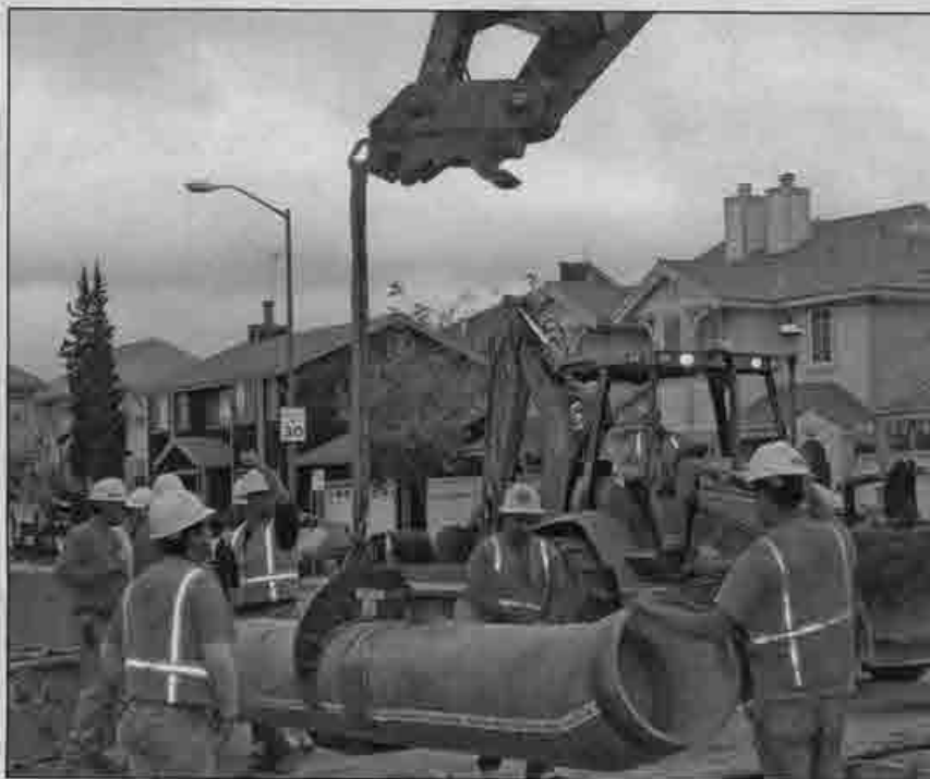
Operating Engineers work with union laborers, welders, pipefitters and sawcutters to ensure the pipe is level and set into the right position underground.
