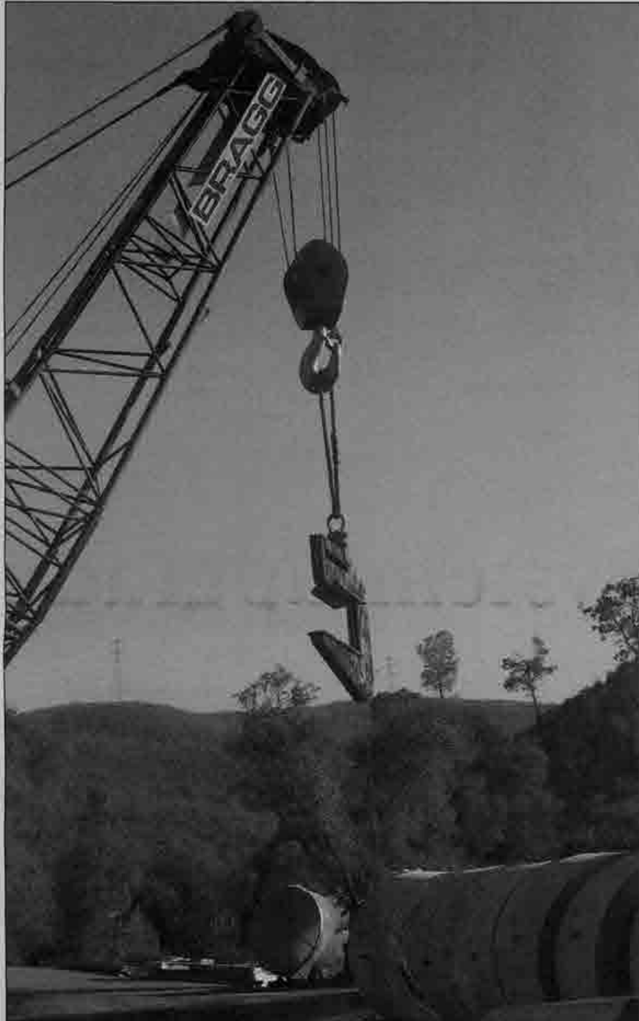
Three Bragg cranes are used at the Priest Reservoir site to move sections of concrete pipe.
