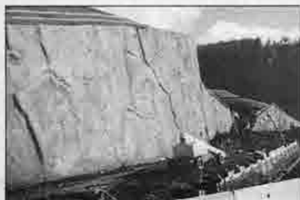
When completed, the Hwy. 101 slide repair project will boast the biggest soil nail wall on the West coast.
