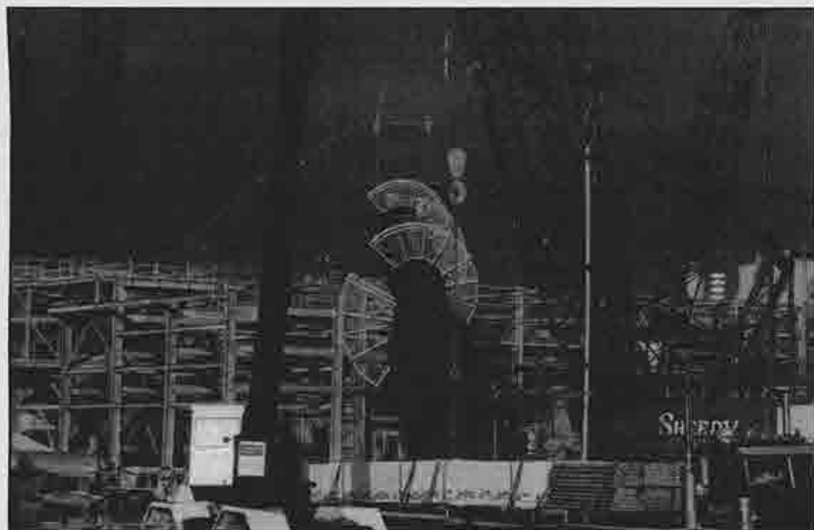
◀ Lift of the delayed gas hydro treater (DGHT) fractionation column at the Shell Oil Refinery.
