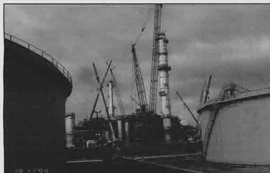
◀ Lift of decyclohexanizer (DCH) column at the Shell Oil Refinery.
