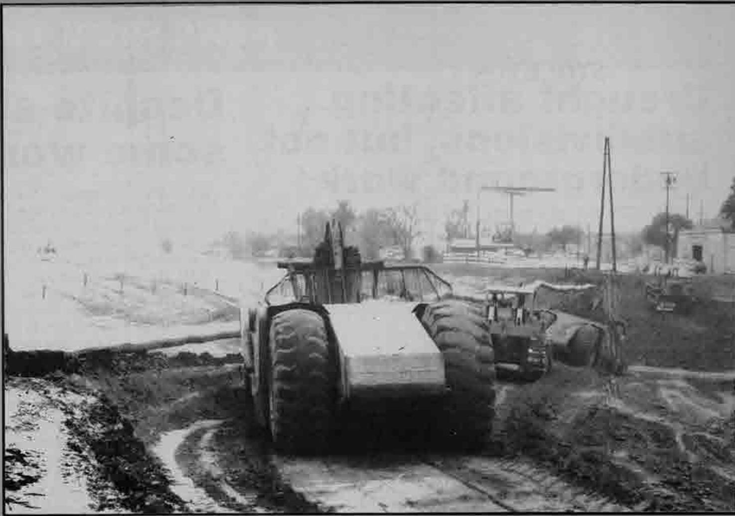
Three quarters of the two-mile section will be built below ground level; requiring about 800,000 cubic yards of excavation.
