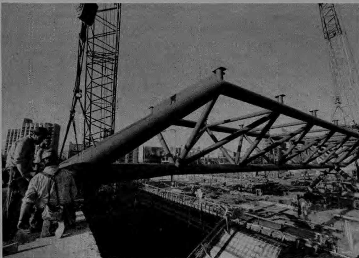
Working off one signalman, two Local 3 crane operators set the massive truss in place while iron workers secure it.
