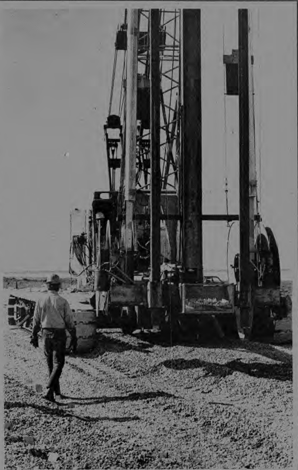
Fast working polyvinyl dewatering wicks are installed deep into the swampy ground with a pile driver. The wicks shorten the drainage period by up to 60 years. Average settlement of the soil is expected to be 4 ft.
