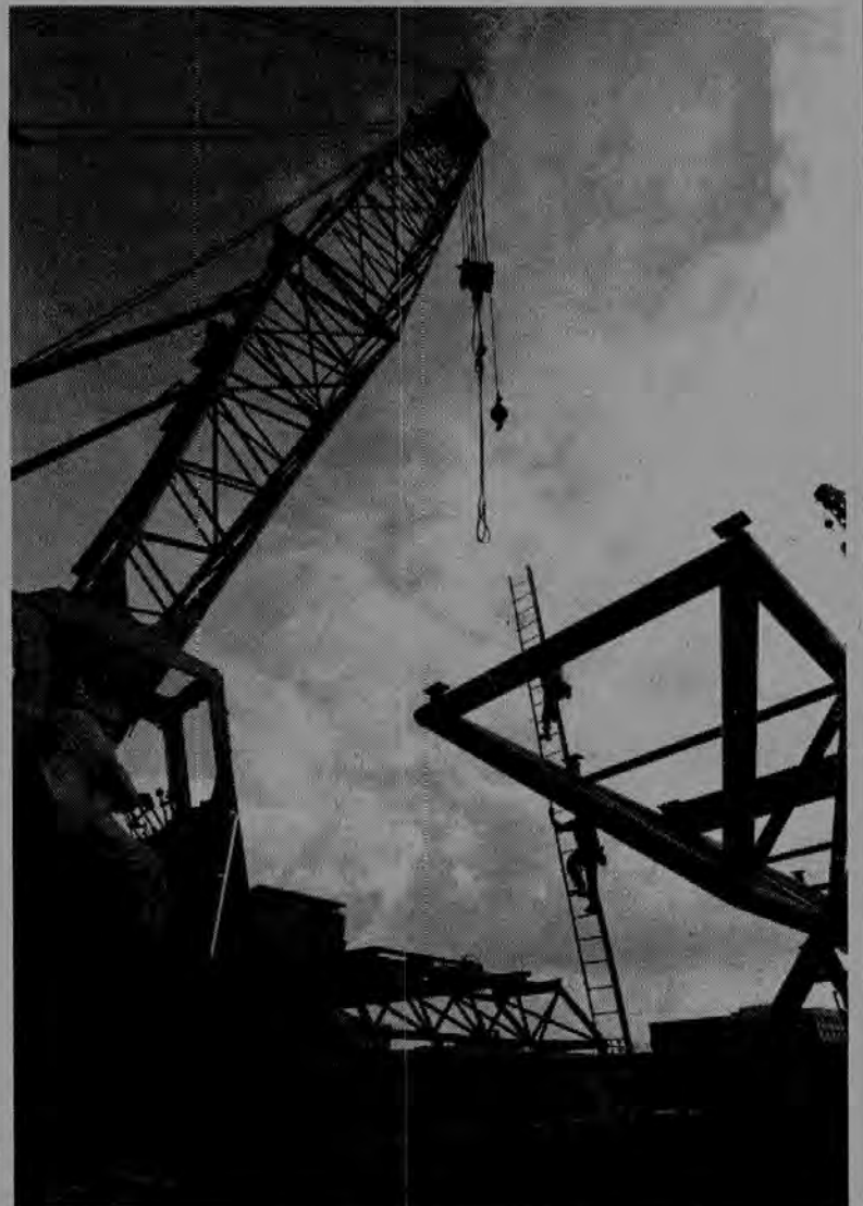
Working off one signalman, two Local 3 crane operators set the massive truss in place while iron workers secure it.
