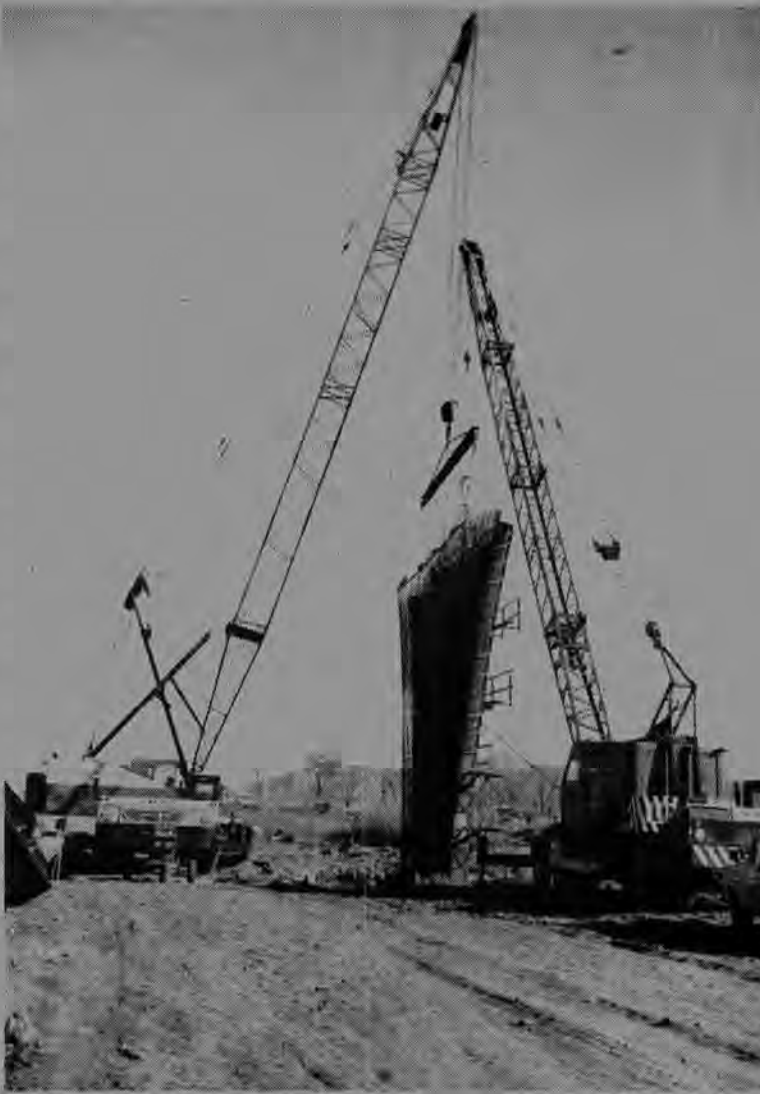
Max Riggs Construction is pictured here building a pier to one of several overpasses on a railroad relocation job near Elko.
