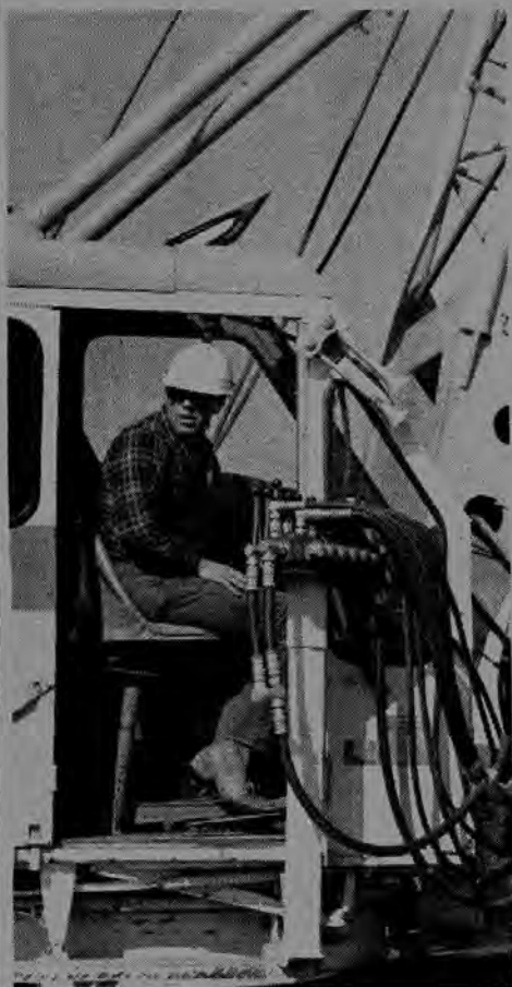
Local 3 member Dan Landis, an employee of Malcolm Drilling Co., operates the pile driver used in installing the unique wick drains.
