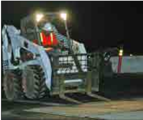
Member George Mejorado uses a bobcat to cover Hwy 99 with 3/4-inch steel plate.
