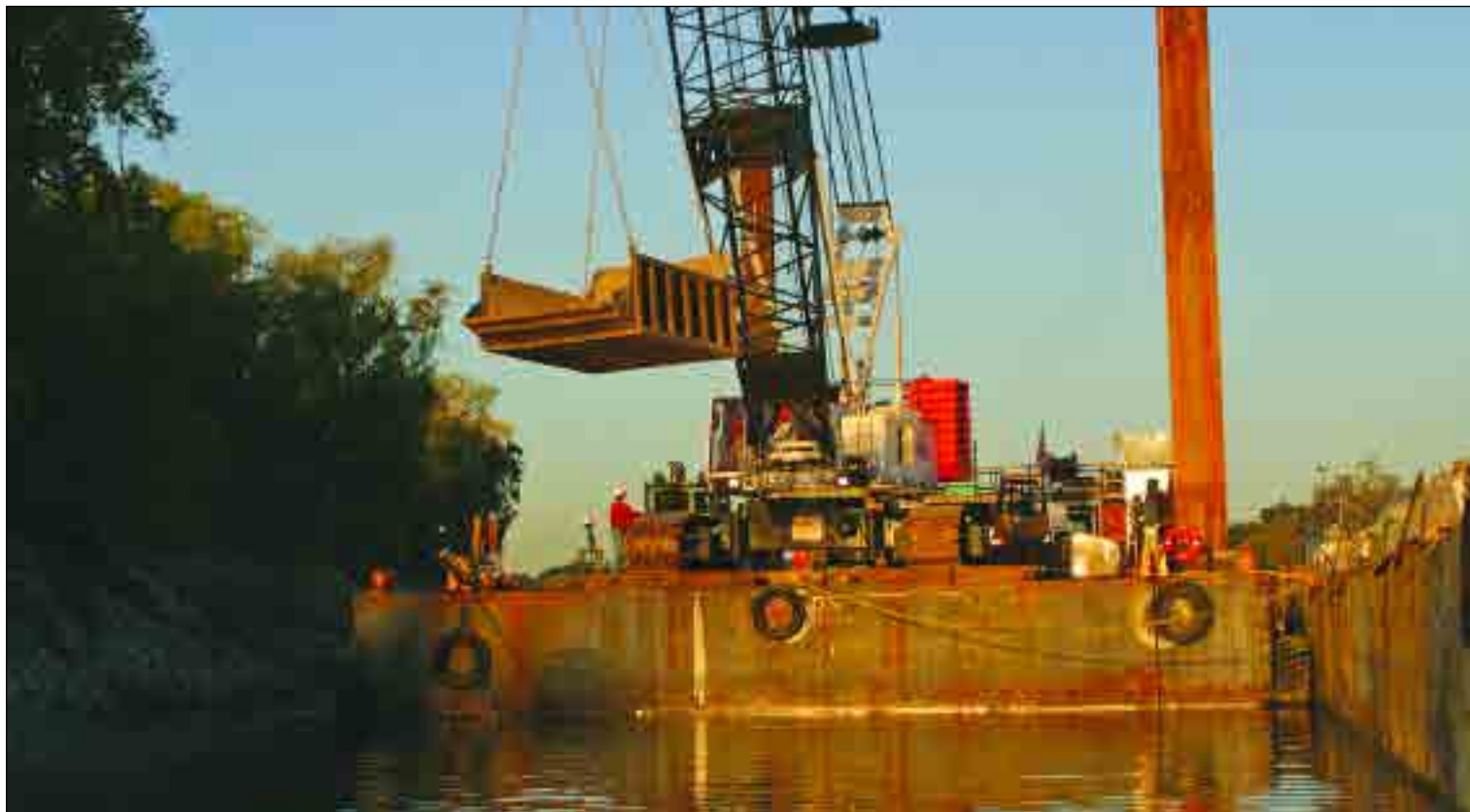
Along the Sacramento River off of Garden Highway, OE3 members Les Darbison and Mike Bledsoe work together to drop aggregate from a barge to the hillside to keep the subdivision overhead safe from flooding.
