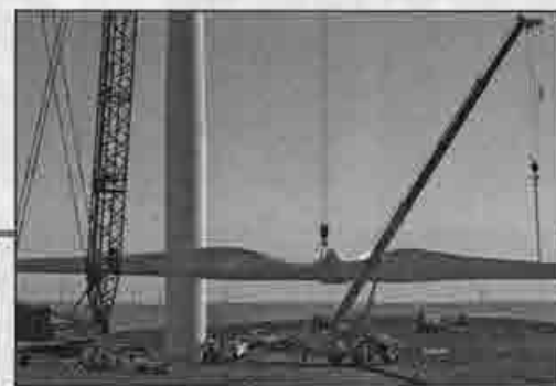
INSIDE: Crane Operators Garth Ungerman and Paul Wright work together to lift a rotor to the top of a wind turbine tower in the Montezuma Hills. 12
