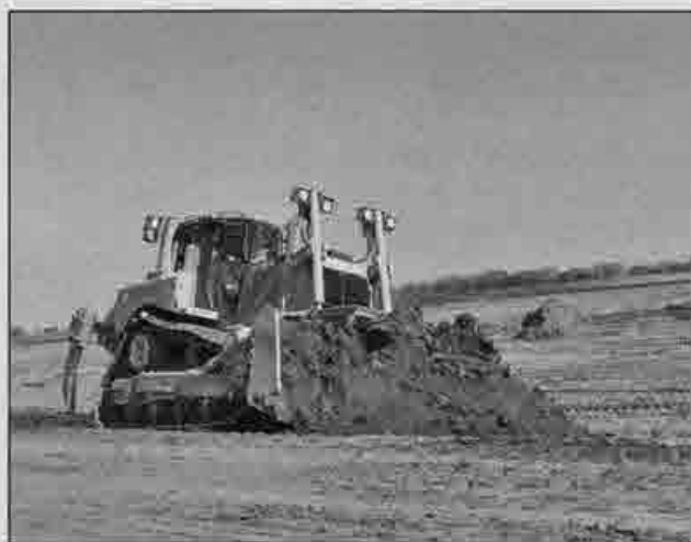
Many dozers work on the River Islands at Lathrop project to create temporary levees in phase one.
