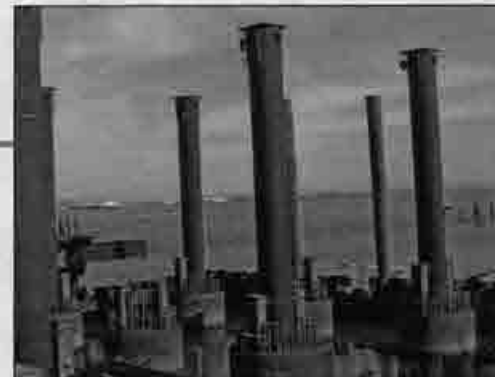
Piling and rebar are locked into place in Cast in Drill Hole casings. .... 11
