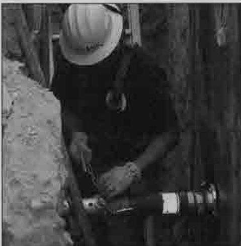
A firefighter sets an air-shore device to prevent a trench collapse.
