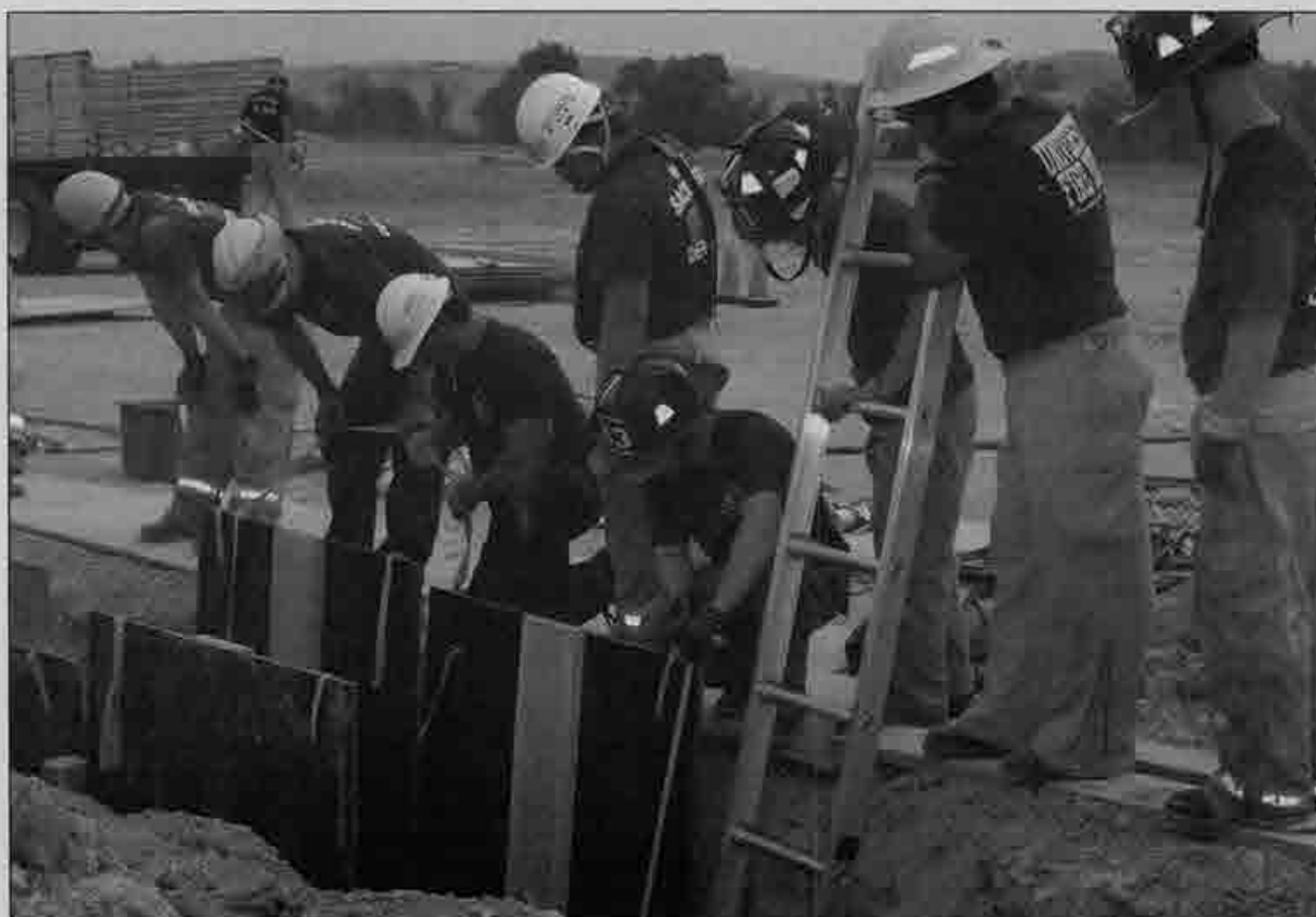
With the walls of the trench secure, firefighters guide and support their teammates working from the ground below.
