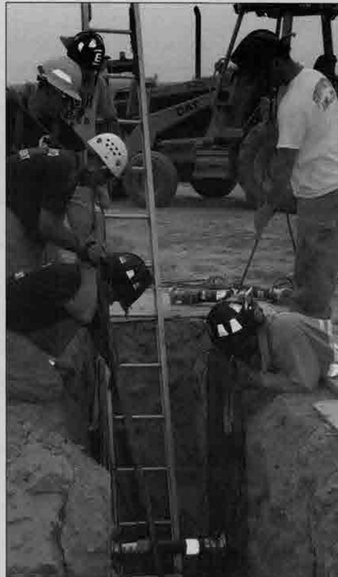
Firefighters work together to shore up a section of a T-trench.
