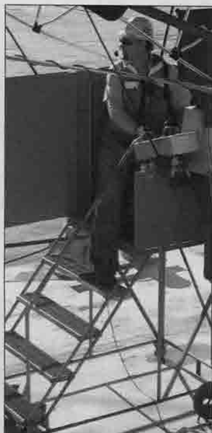
Lee Heidrick operates a wench on the Catamaran Barge to lower a platform into place.
