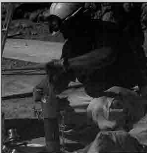
A firefighter readies the air-shore device used to secure the walls of a trench.
