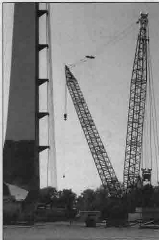
The 217-foot pylon, seen at left, will have 14 cables extending from it to help support the deck structure.
