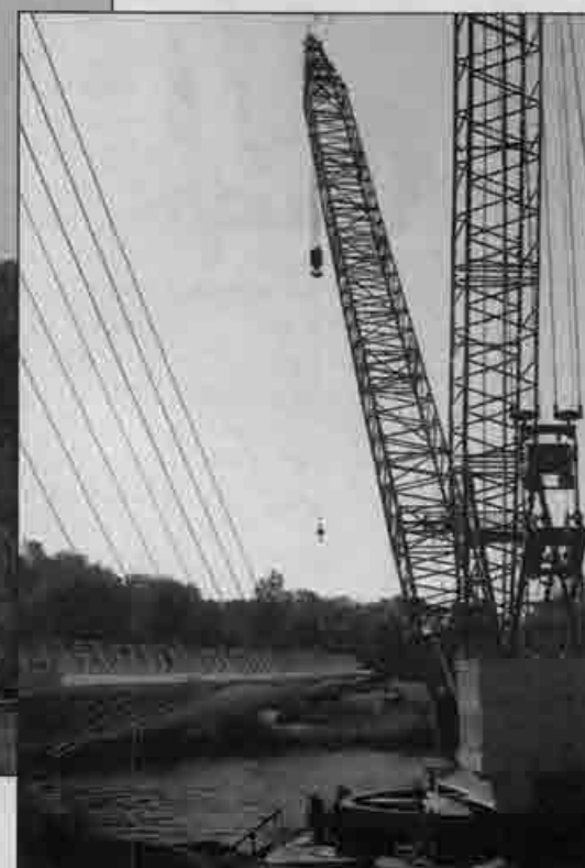
At left will function as a sundial when the bridge is completed. The deck structure is being built from either side of the river, and in the middle. At right: The 300-ton Manitowoc 4100 crane is used to set the pieces of the truss in place.
