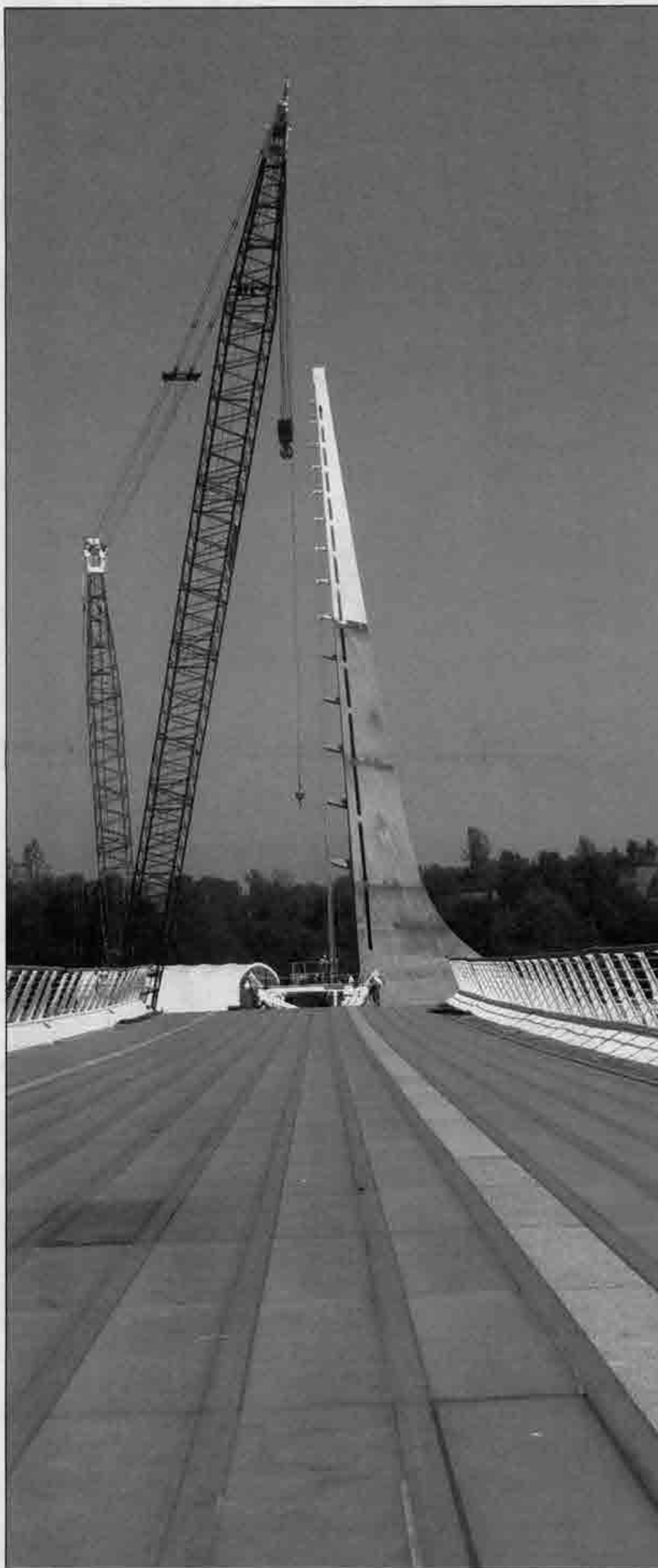
The Sundial Bridge will be asymmetrical with the pylon on one side and 14 cables that will extend from that same side. The deck is made of sandblasted glass, granite and steel.
