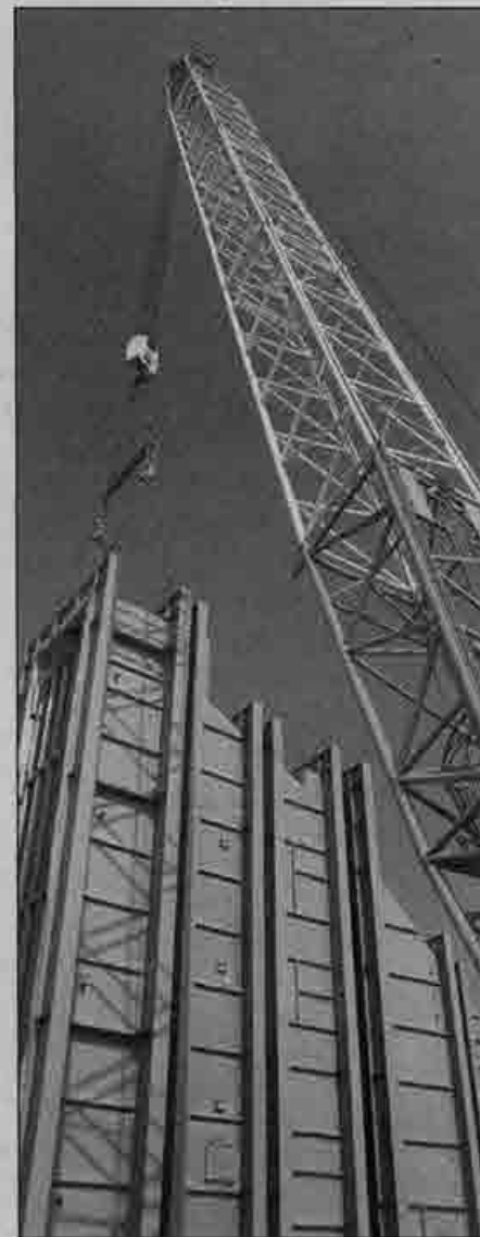
A Demag CC1800 holds a section of the heat generating unit in place.
