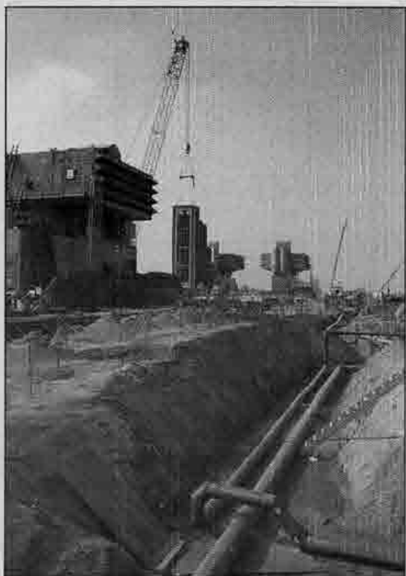
Underground pipes lead to the heat generating units at the Calpine project.
