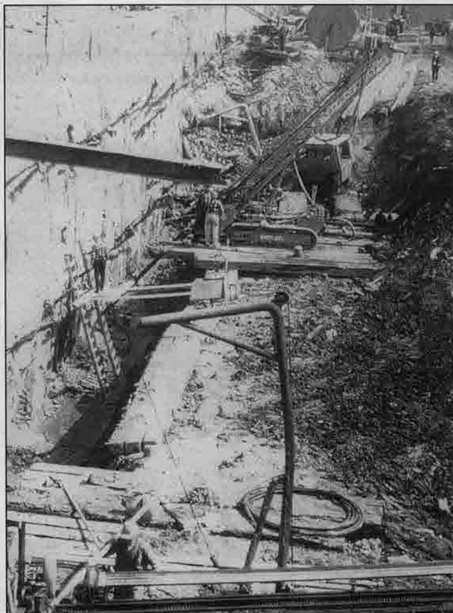
This shows the arrangement for drilling of tiebacks at Vesey Street, where second-level tiebacks are being drilled. This is necessary if the walls are to be resupported by tiebacks.
