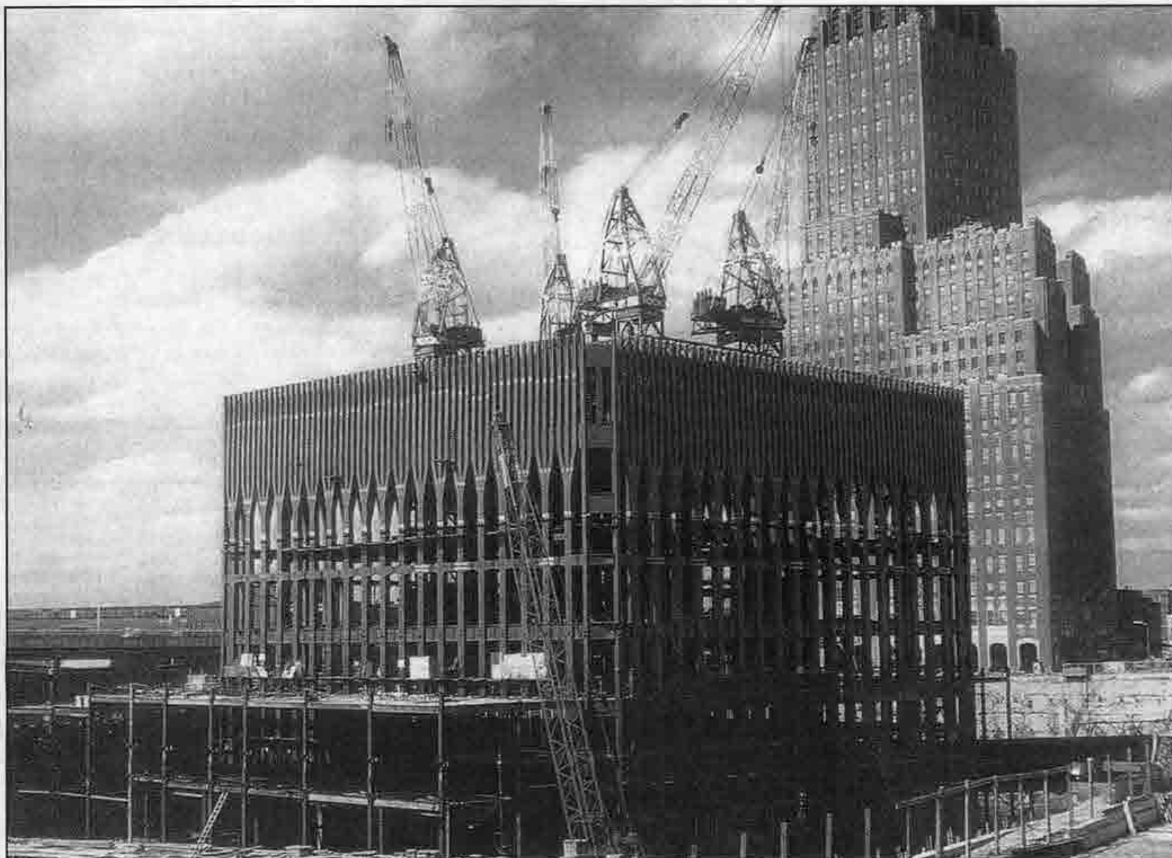
Yokes and typical fascia framing for the steel for Tower No. 1.
