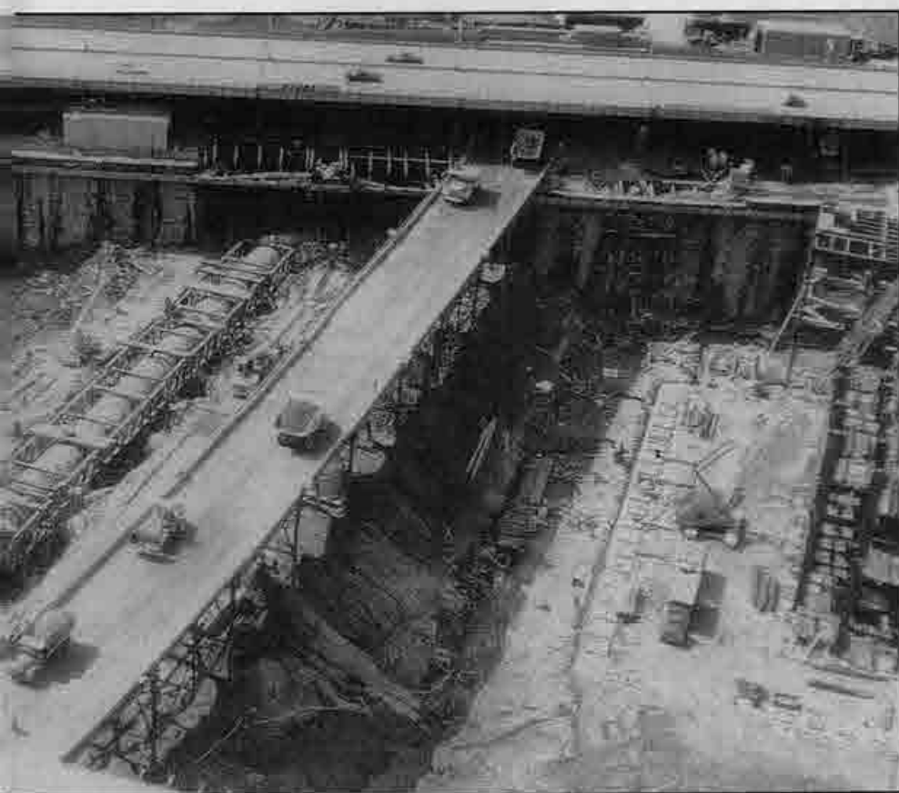
Left is the SW corner of the WTC Complex at Liberty and West streets. The PATH tube, which has been removed, is shown diagonally across the photo. Next is the temporary construction bridge used for trucks to haul excavated material out of the site. To the right is the beginning of the erection of steel for the No. 1 (North tower).
