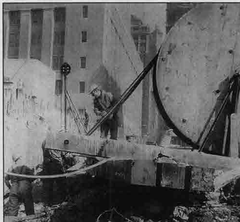
Installation of the tieback tendons.
