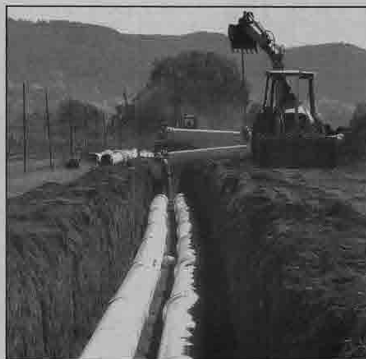
DUAL PIPES: Local 3 operator Dave Wilson lays dual pipes.
