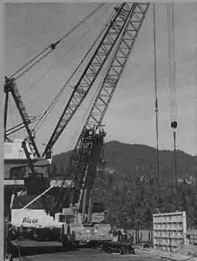
A Fletcher General's gantry crane and Bigge's hydraulic crane team up to lower one of the steel gates into the water.
