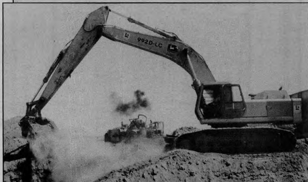
Below: A backhoe from Floyd Johnston Construction over excavates in preparation for recompaction.
