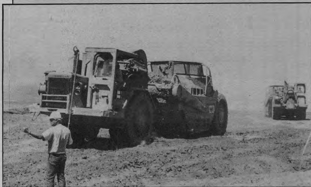
Above: Scraper operators move some of the project's 1.7 million yards of dirt.
