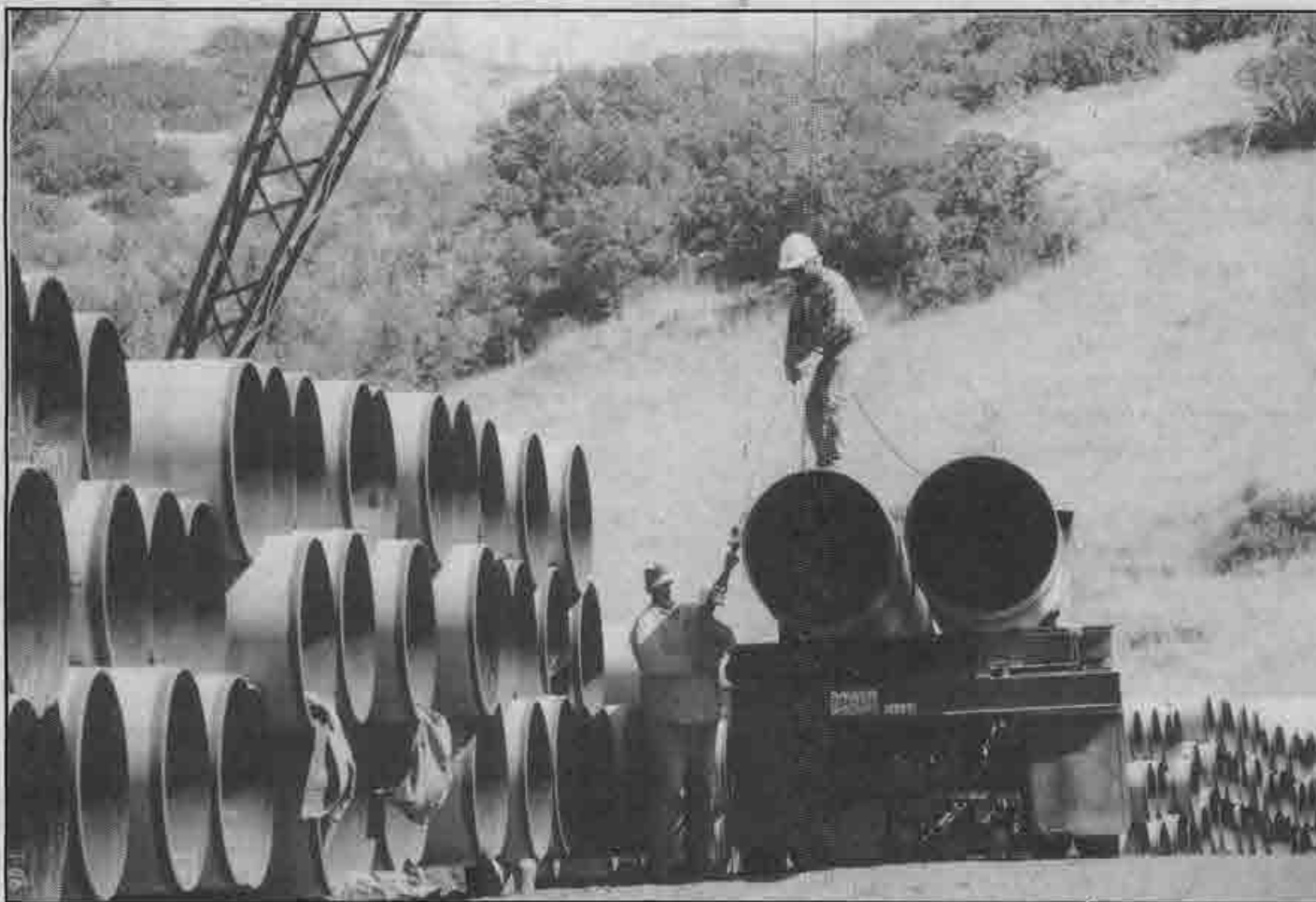
Laborers working for Associated Pipeline (left) prepare to unload a truckload of 36-inch pipe to be used on the Kern River Gas Transmission pipeline. The crane operator working on this crew is Gordon Ferguson (above left), a 43-year member of Local 3. He is assisted by oiler Chuck Valdez.
