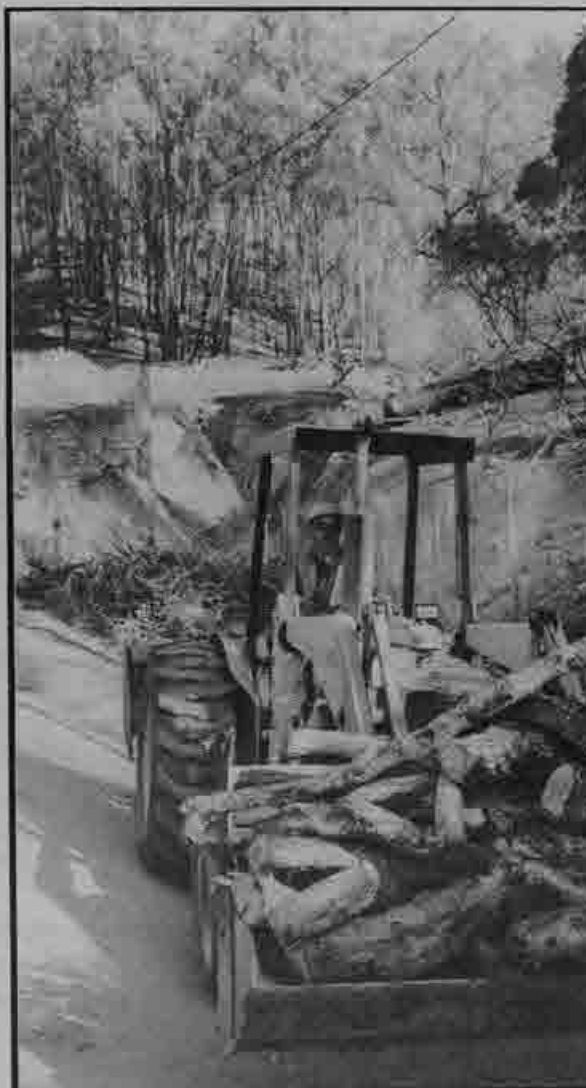
Top and center left: Miguel Pineda and Dave Lehman clear burned vegetation above Caldecot: Tunnel before winter runoff causes debris to clog storm drains.
