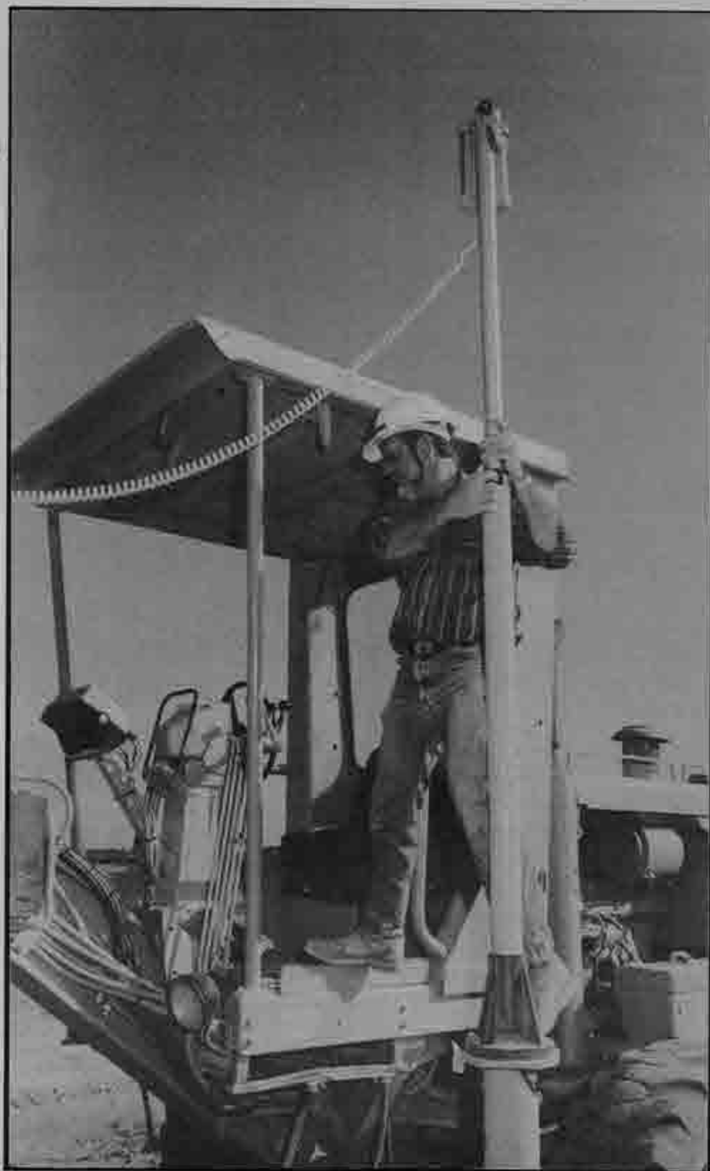
Below right: Blade instructor Tom Mullahey watches the lights on the control panel of laser device as he adjusts the mast with sensor atop.
