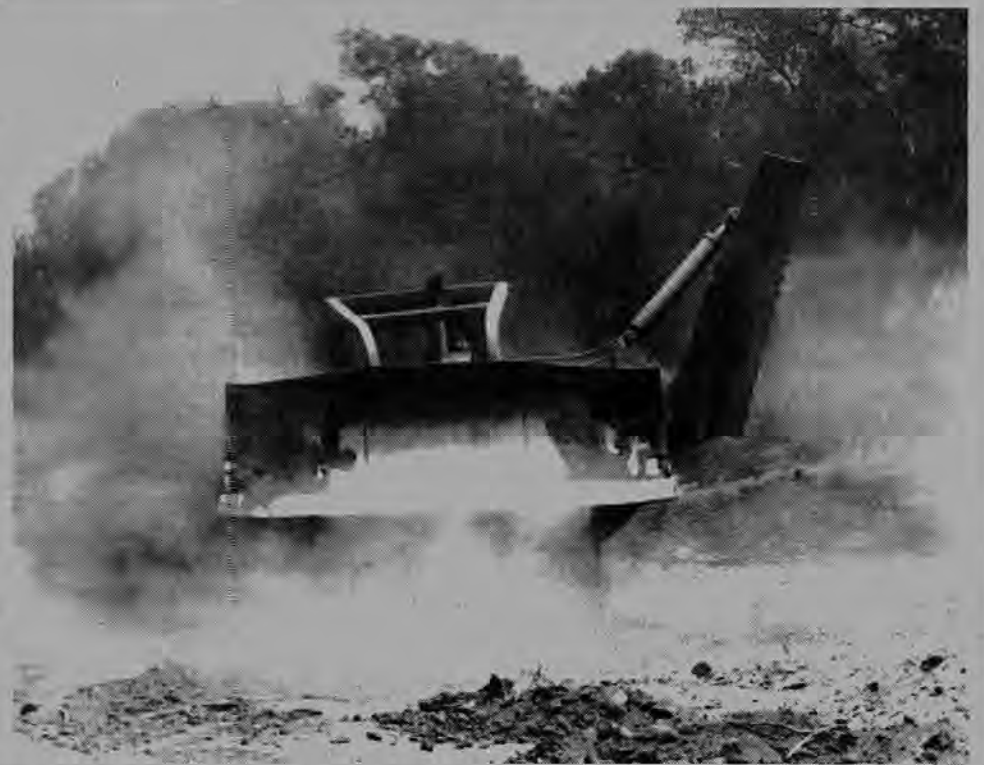
Local 3 member Art Wisterman operates this dozer mounted with slope board on the Fountain Grove Expressway project in Santa Rosa.
