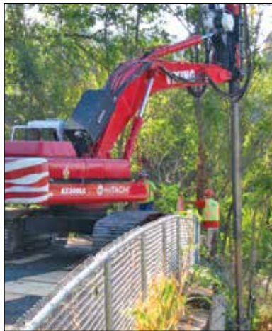
Working for Viking Drillers, members Erik Bakken and Jose Arellano work in District 30 repairing a retaining wall.
