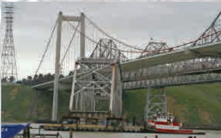
As soon as the first section of deck is down, a tugboat hauls it away from the bridge, beginning the first of many treks to Mare Island.
