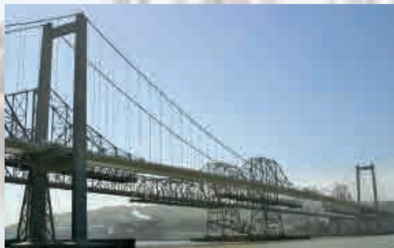
A second deck section is removed from the bridge May 11. Each section weighs 700 tons and is more than 400 feet long.
