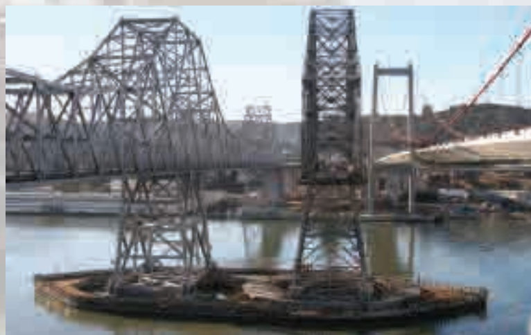
Local 3 members built platforms to dismantle the bridge piece by piece.
