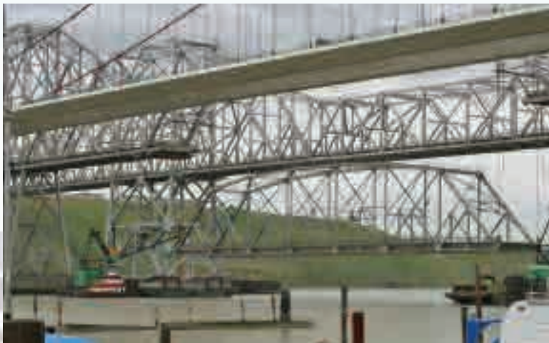
Using four strand jacks (for a total of 76 strands), operators begin the Carquinez Bridge demolition by lowering the first section of deck.
