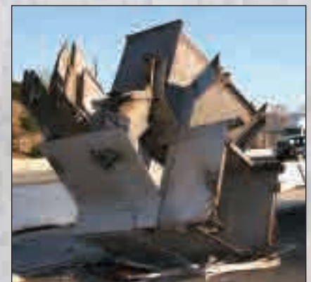
These giant knuckles are like hinges holding the pieces of the old Carquinez Bridge together and are just one of the many parts deconstructed. These will be used as historical items in area museums.
