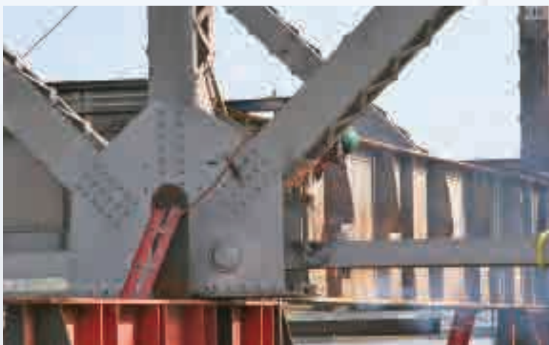
OE3 members torch the remains of the 1927 Carquinez bridge, and the remains are used as scrap metal at Mare Island in Fairfield, Calif.
