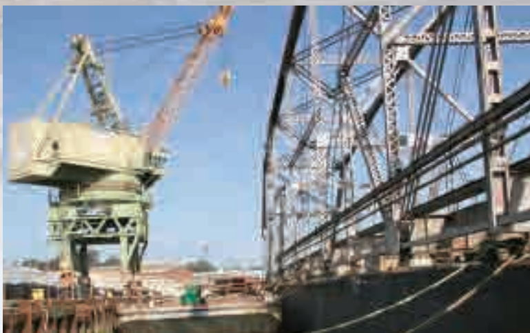
This Washington D7 gantry crane is operated by Local 3 member Vinnie Capizzo, who unloads pieces of the 1927 Carquinez bridge.
