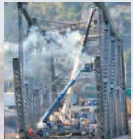
From the northside, a crane is viewed placing pieces of the bridge onto trucks.
