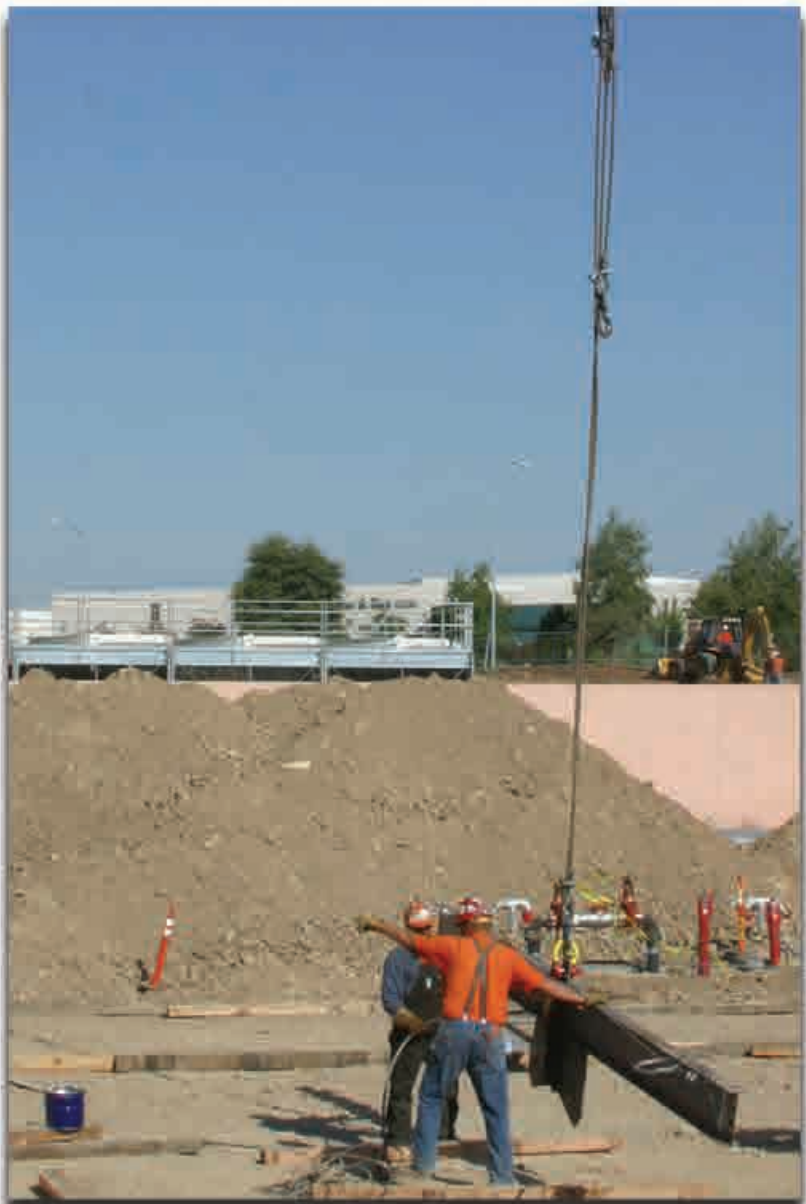
Iron is attached and hoisted to the penthouse of the building.
